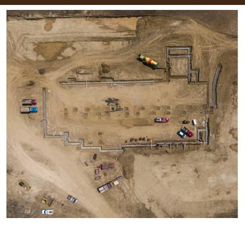
New facility update: Woodridge is excited to share an update about Phase 1 of the construction project. Crews are hard at work installing water mains, underground plumbing, building geothermal wells, and more. For more information about the project, please visit the Woodridge New Facility Needs website.
