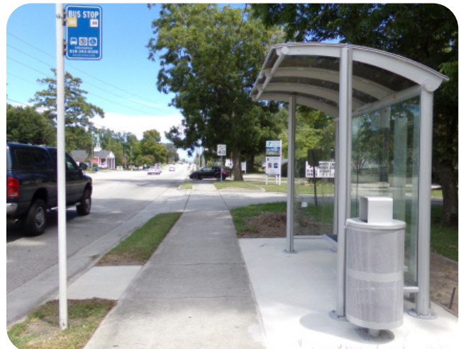
ELKWOOD AVENUE @ MERRIMON AVENUE
