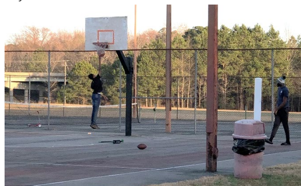
Camptown Park – aging furnishing and basketball court needs resurfacing
