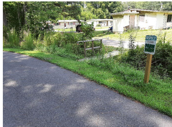
Park – to – Park asphalt trail with a detached bridge to allow adjacent community to enter.
