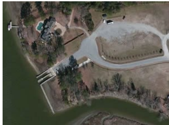
Jones Creek Boat Ramp aerial photo
