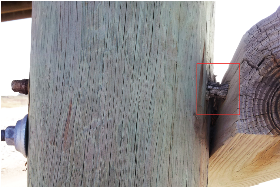
Photo 3. The old bolt is severely corroded and reduced in diameter compared with the newer stainless steel bolt below.
