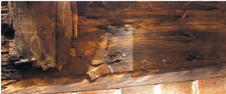
Photo 4. Inadequate flashing contributed to the decay of this band joist where a deck ledger was connected. No quantity of fasteners will secure a deck to this band joist.
