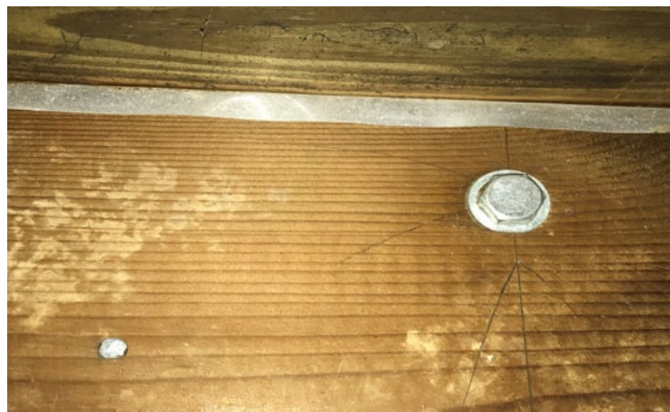
Figure 2. Section of a deck ledger with a nail head and ½" diameter lag screw installed.
