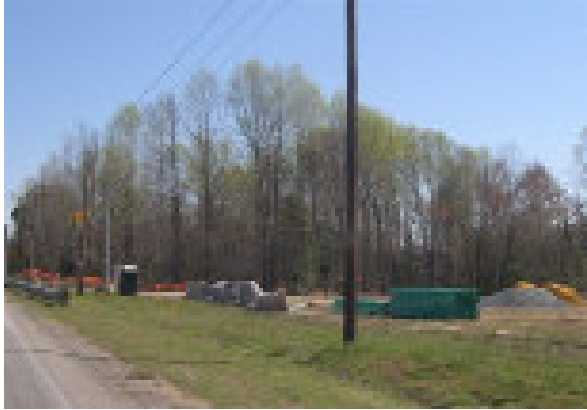
Onsite drainage materials
