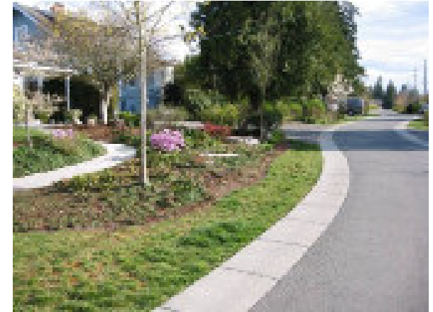
Swales, narrow pavement, flat road edges instead of curbs, and landscaped rain gardens are characteristic of low-impact development.
