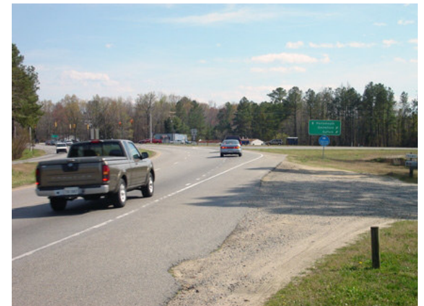
Route 17 and 32 Intersection
