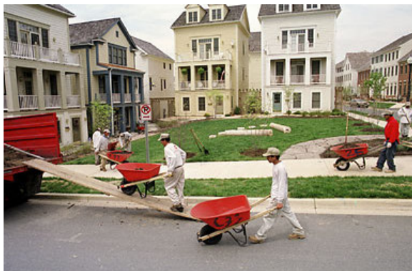
A TND under construction
