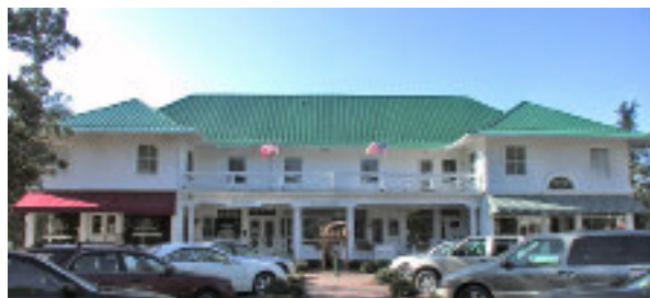
This is a good example of 2-story mixed use building, with a range of desirable vernacular forms and materials. The placement, however, of a parking lot directly in front of the building should be avoided.
