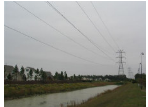
Overhead power lines
