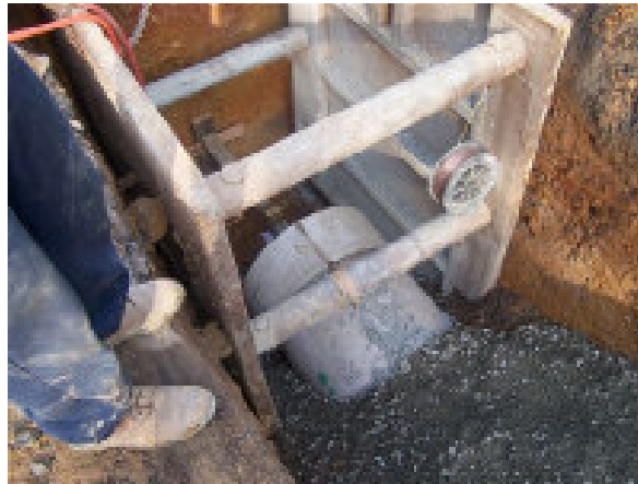
In-ground utilities construction
