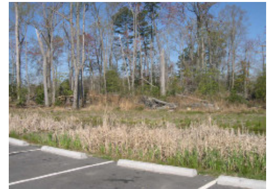
Stormwater management devices serving existing development in the study area
