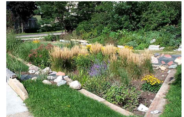
Bioretention Best Management Practice (BMP)
