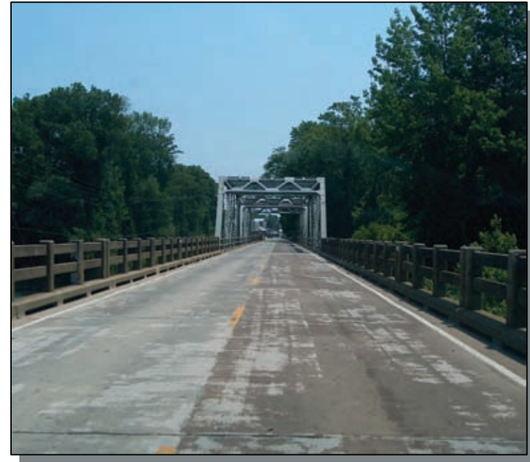
PICTURE 4 – The Route 35 bridge over the Nottoway River in Courtland is classified as functionally obsolete. Functionally obsolete bridges are those bridges that don't meet current design standards.
