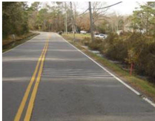
Figure 18. Example Rumble Strips (Source: FHWA)
