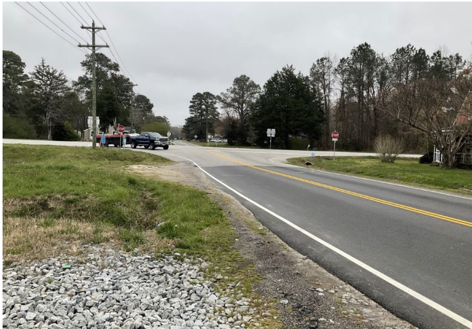
Figure 13. Pavement markings and stop signs without retroreflective element.
