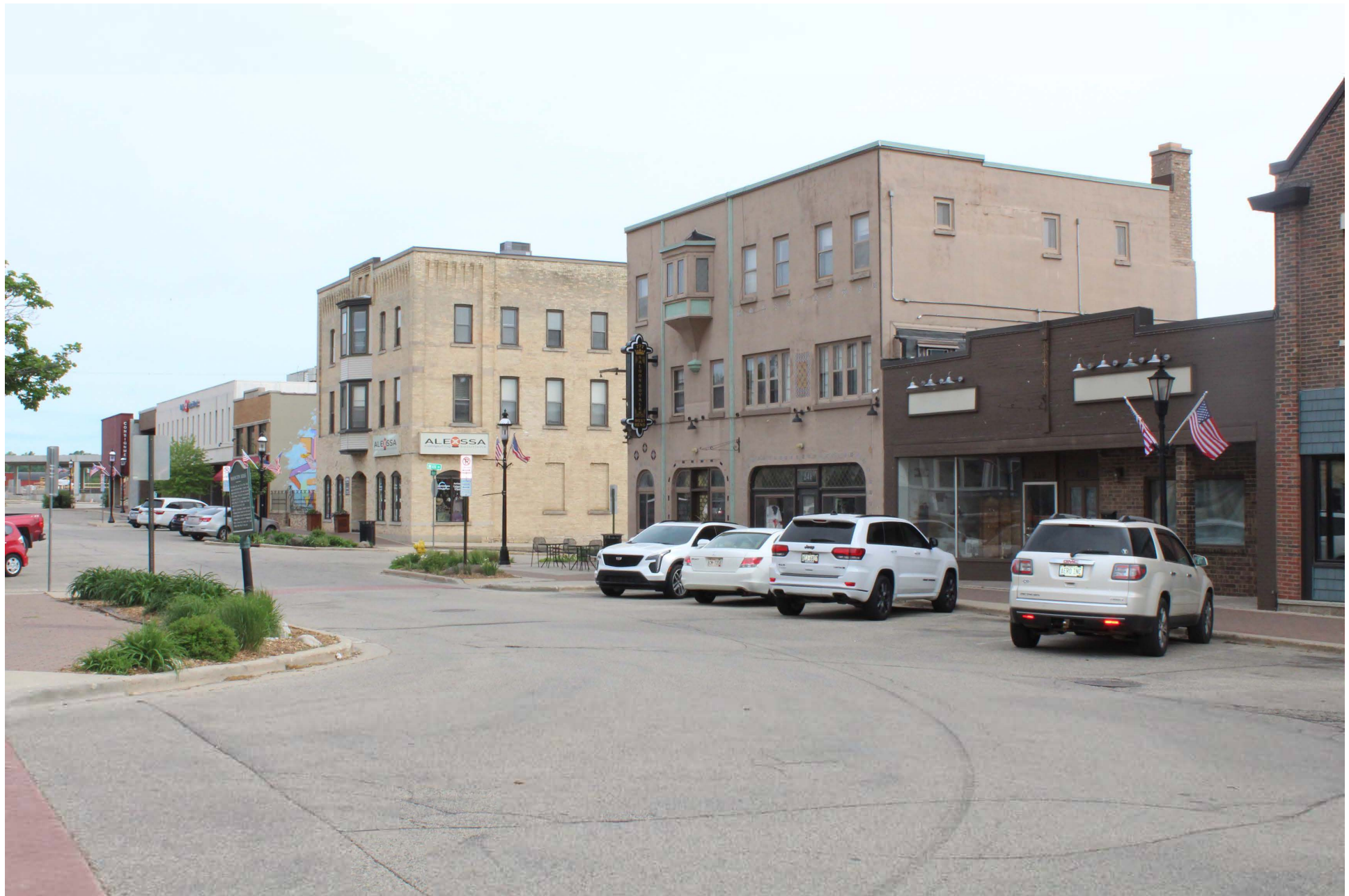
West Bend Downtown Historic District, West Bend, Washington County, 5 of 17
