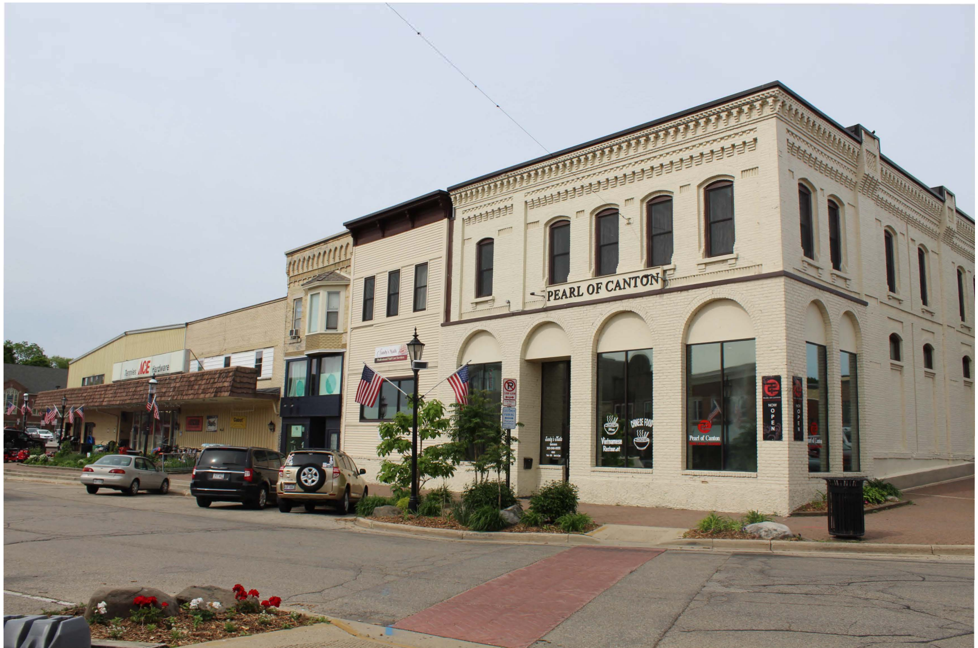
West Bend Downtown Historic District, West Bend, Washington County, 16 of 17
