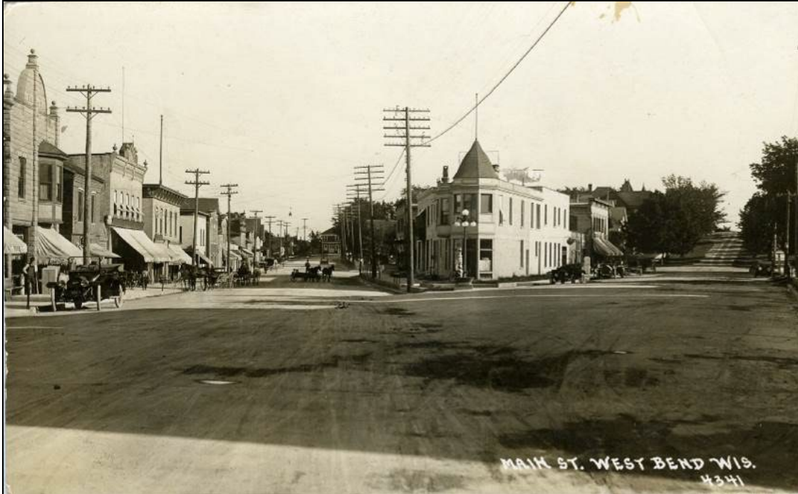
Figure #5: View of South Main Street. 125 South Main Street at far left, 136, 146-156 and 160-162 South Main Street at center. 5 th Avenue is the street at the right (WCHS 015,541; undated but perhaps circa 1920).
