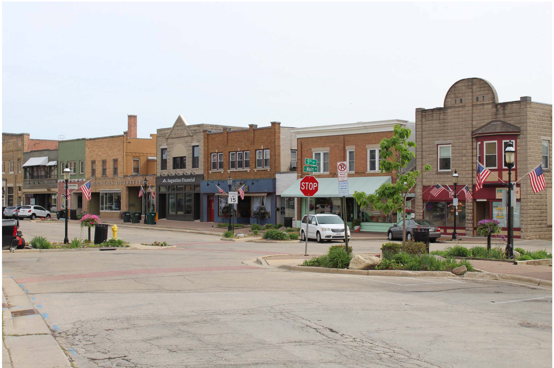
West Bend Downtown Historic District, West Bend, Washington County, 15 of 17
