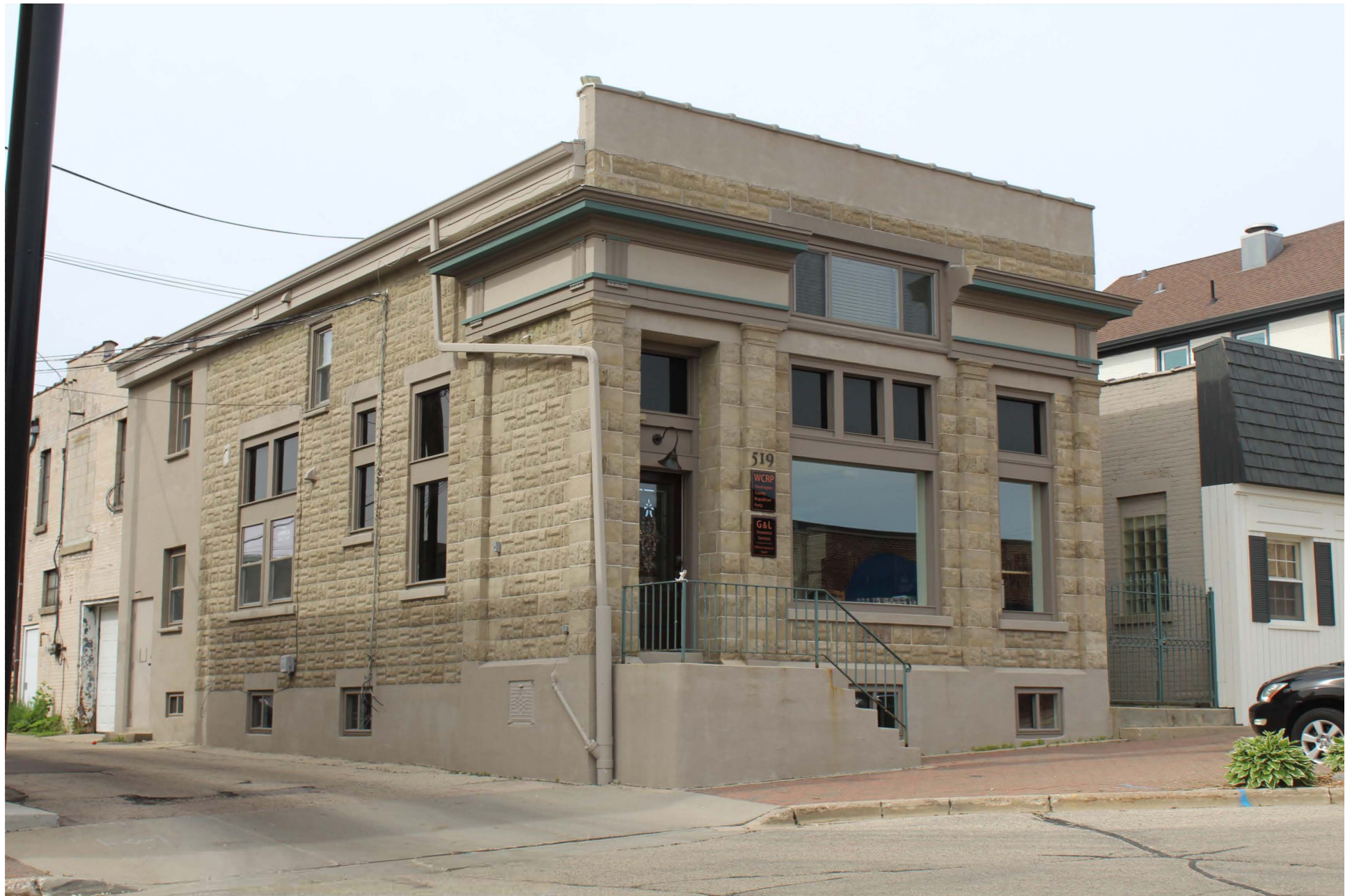
West Bend Downtown Historic District, West Bend, Washington County, 13 of 17
