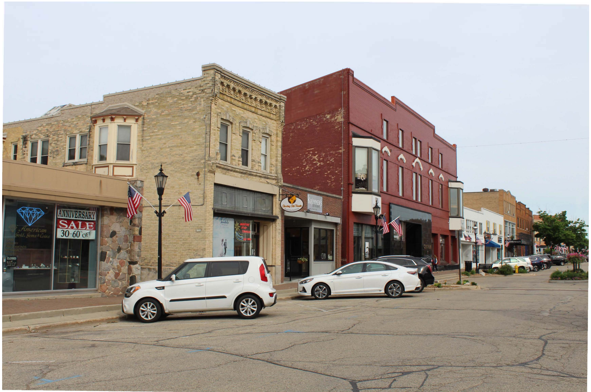
West Bend Downtown Historic District, West Bend, Washington County, 10 of 17
