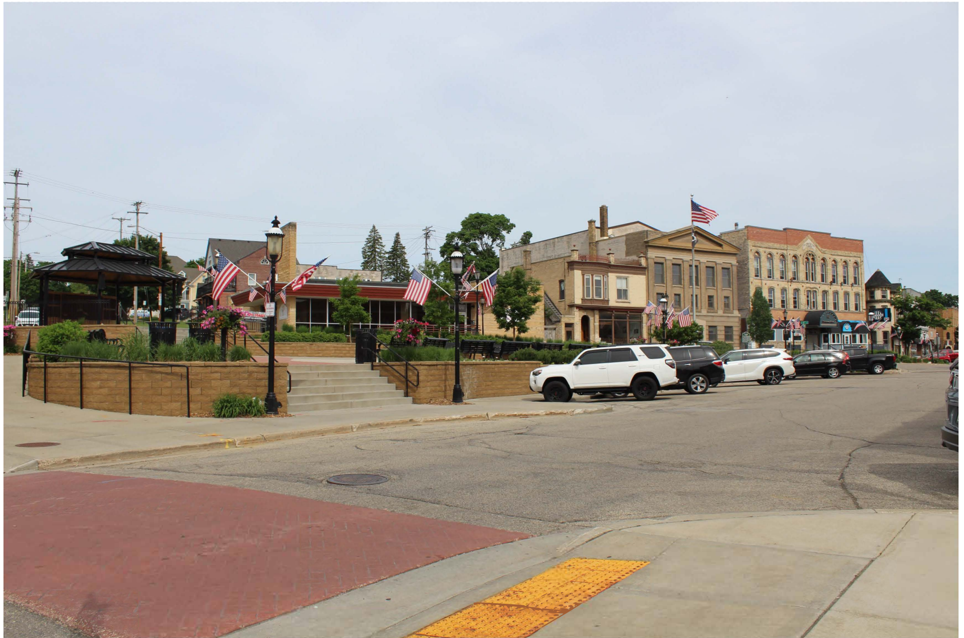
West Bend Downtown Historic District, West Bend, Washington County, 7 of 17
