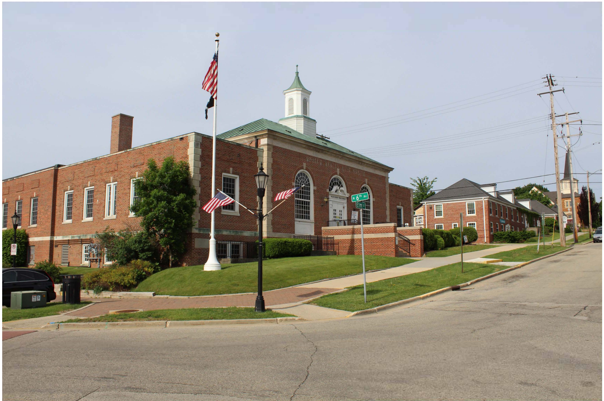
West Bend Downtown Historic District, West Bend, Washington County, 8 of 17
