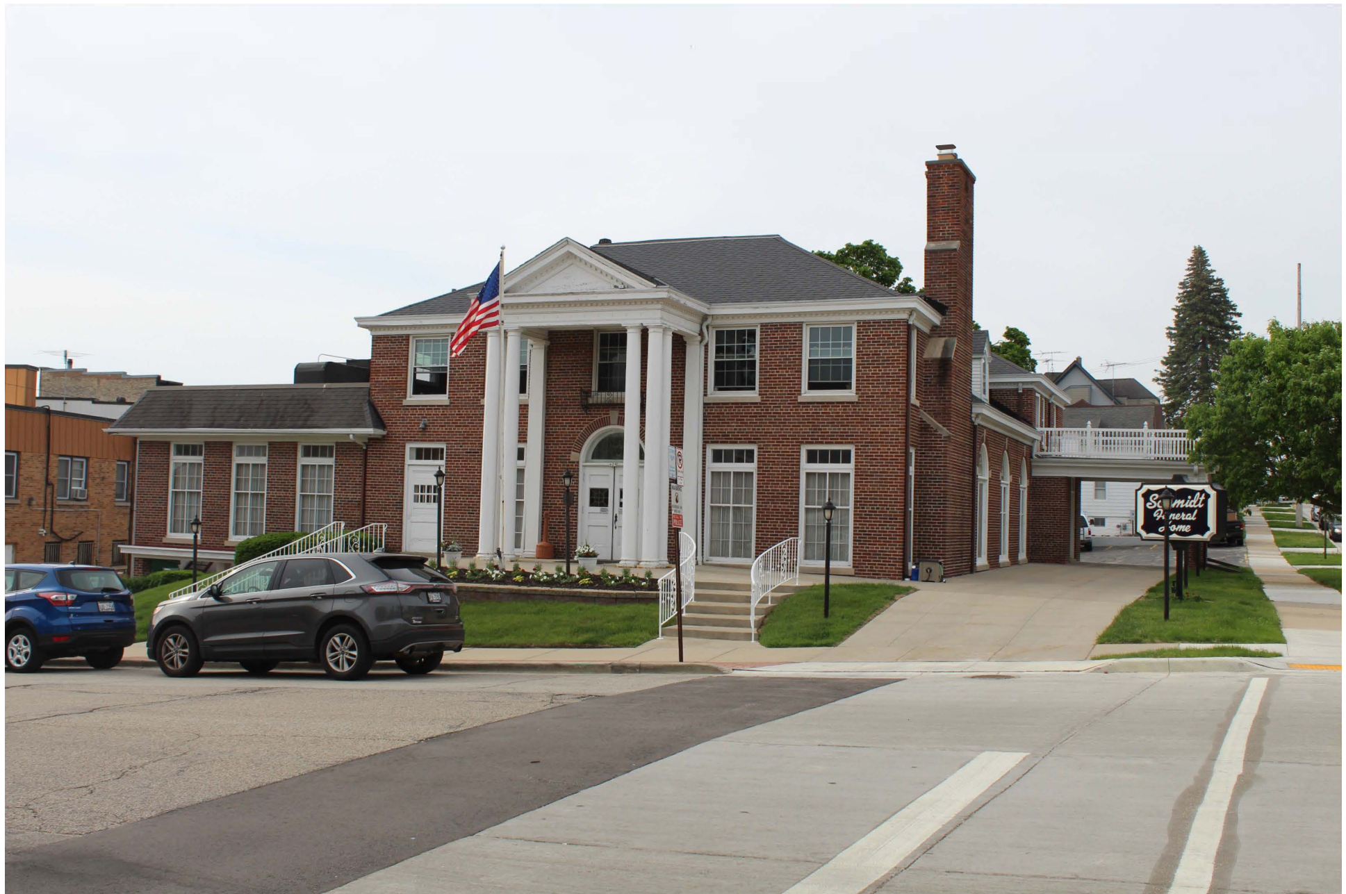
West Bend Downtown Historic District, West Bend, Washington County, 3 of 17
