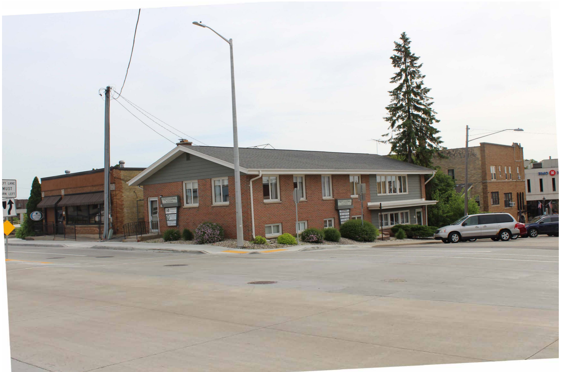
West Bend Downtown Historic District, West Bend, Washington County, 2 of 17
