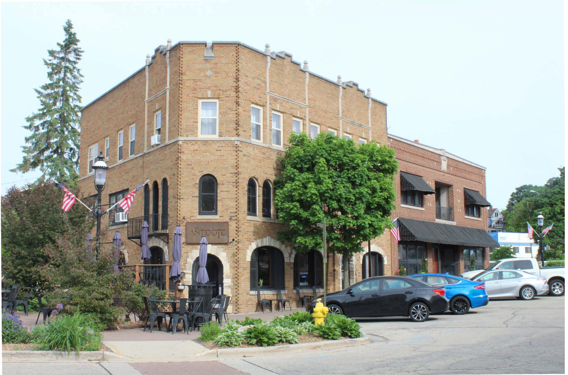
West Bend Downtown Historic District, West Bend, Washington County, 1 of 17
