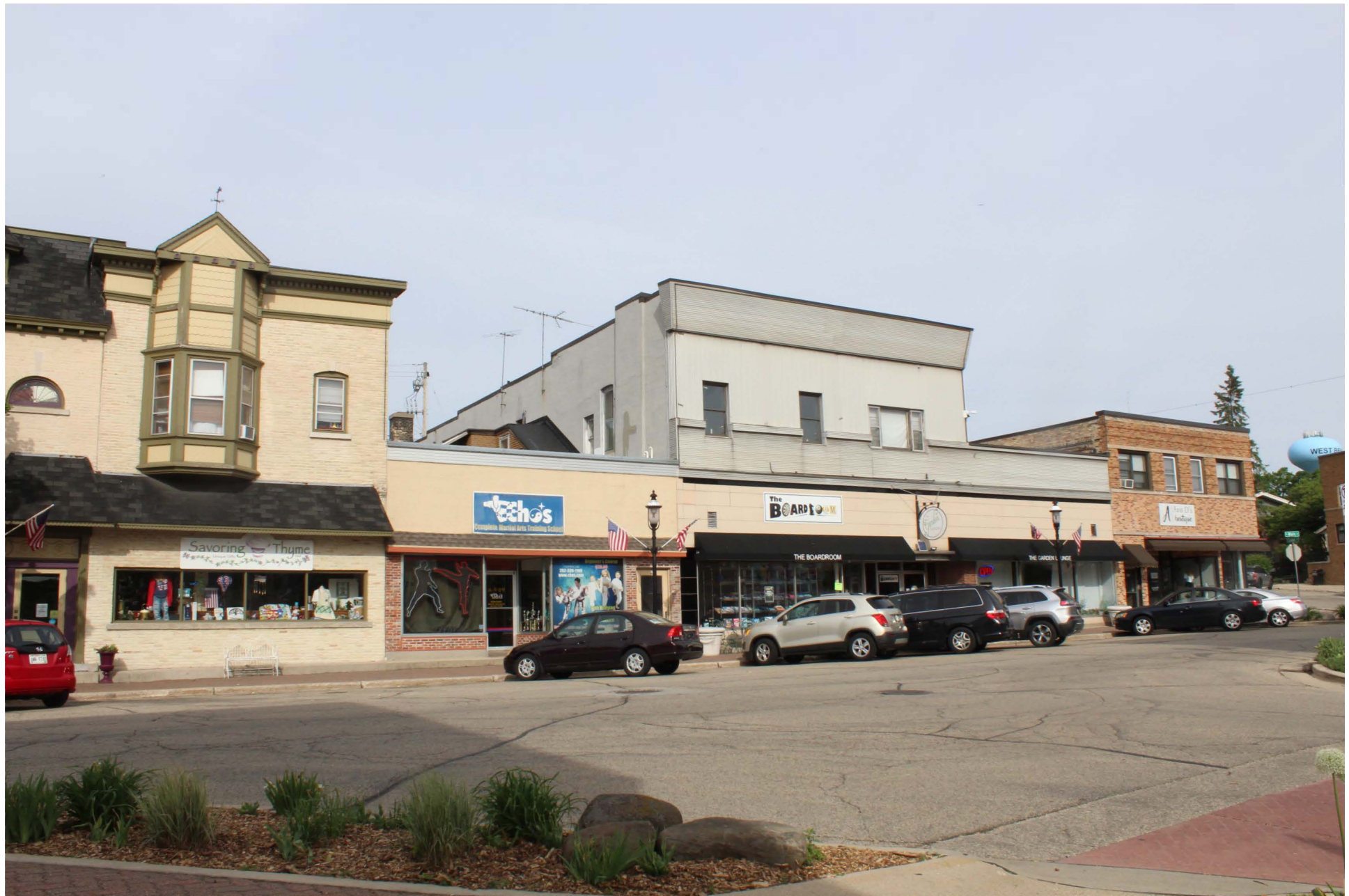
West Bend Downtown Historic District, West Bend, Washington County, 4 of 17
