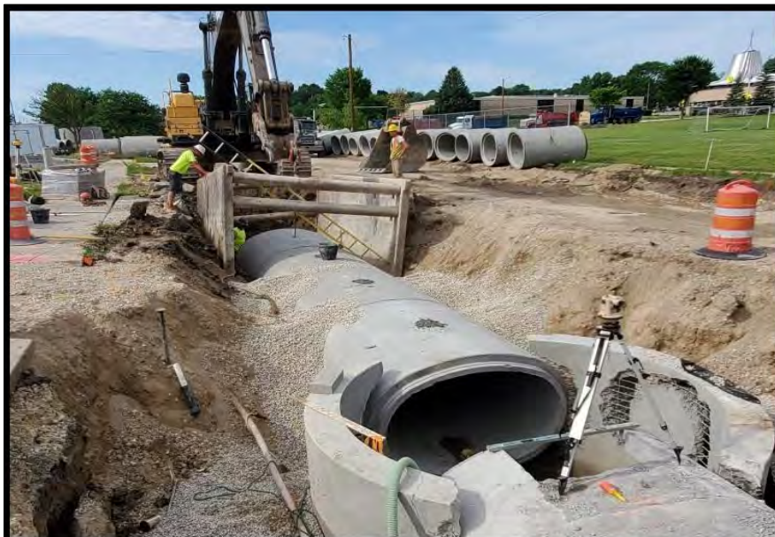
Installation of storm sewer pipe under contract 22-01 (5th Avenue reconstruction; Hawthorn to Decorah)
