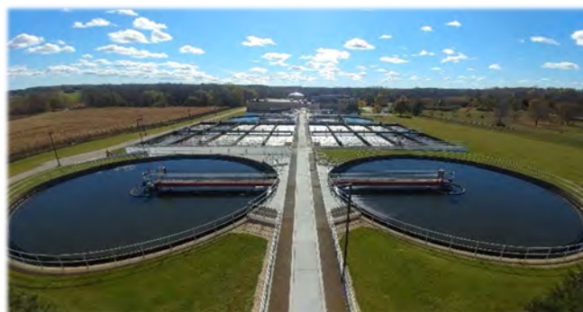
Overhead view from Trickling Filters
