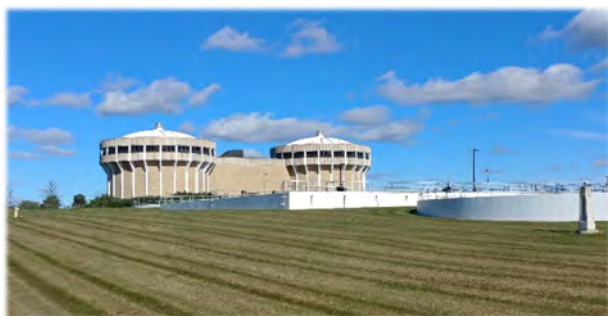
Ground level Trickling Filters
