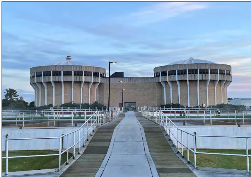
Aeration Bays and Trickling Filter Towers
