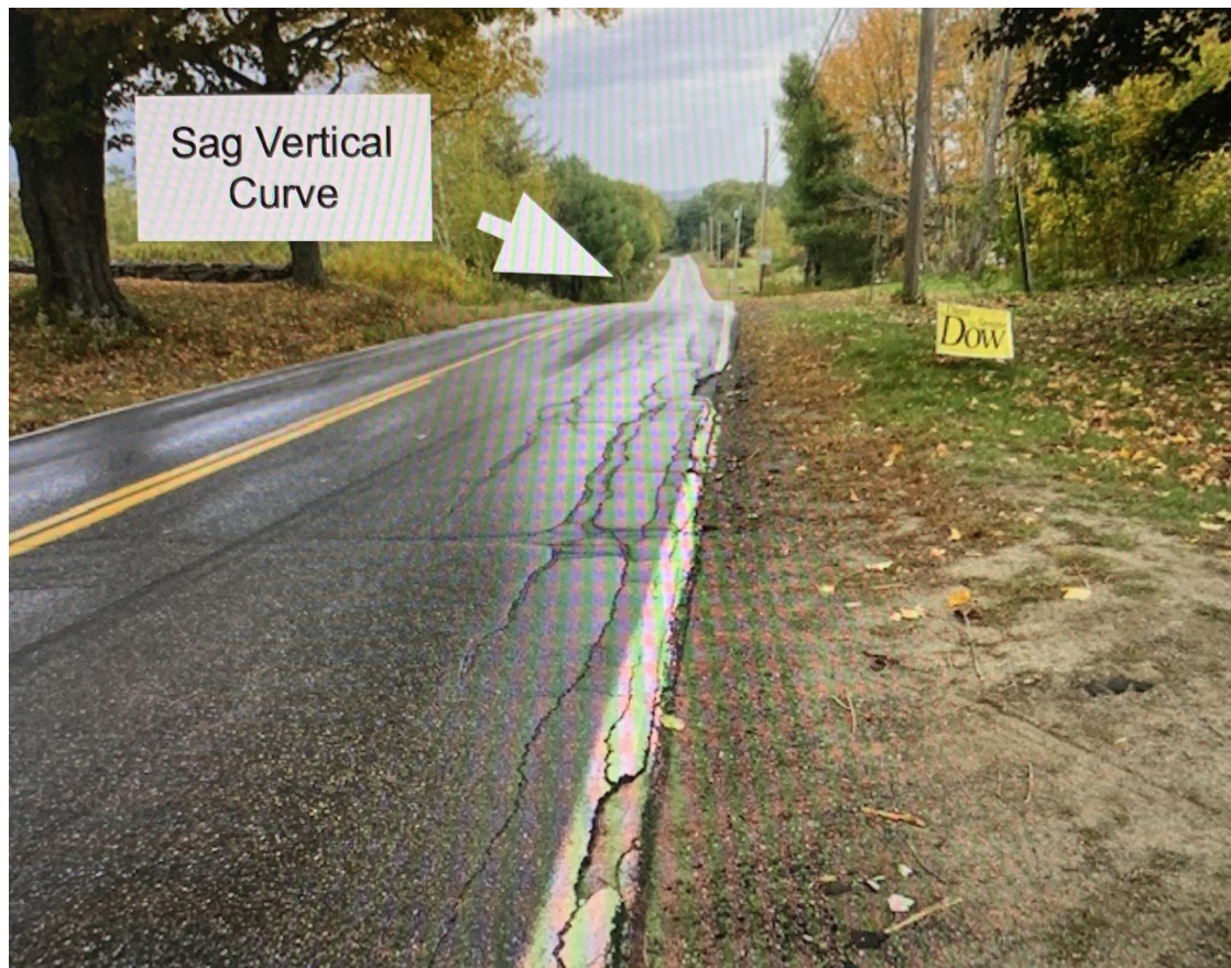
Figure 3.4 Shows the Vertical Sag Curve on Old Augusta Road, SB approach
