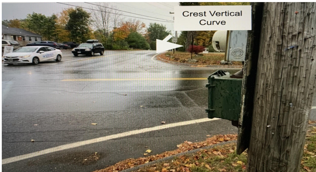
Figure 3.1 Shows the crest vertical curve from SB approach
