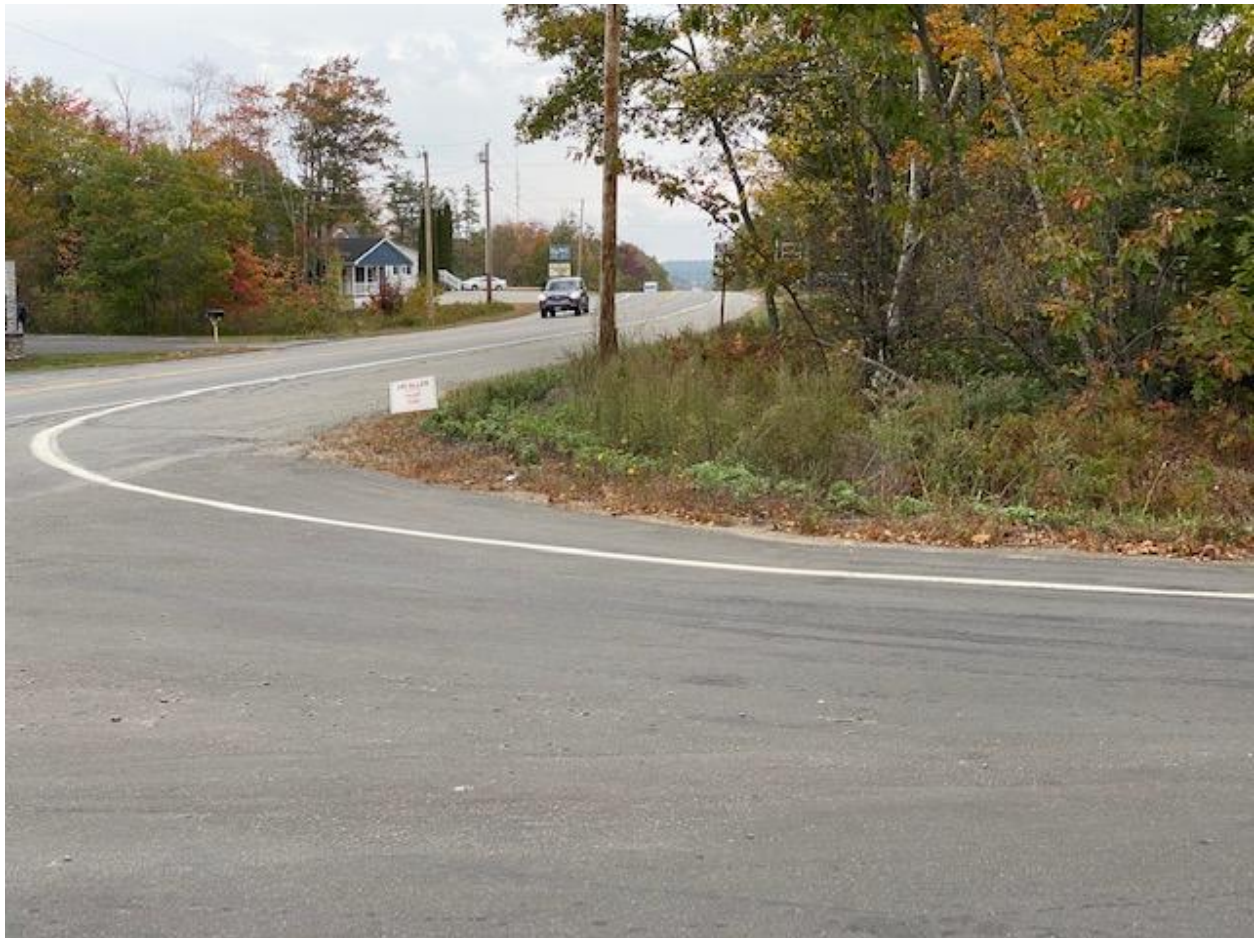
Figure 3.5 Shows Horizontal Sightline obstructions at the Rt. 1 and West Main St. Intersection looking East (right from turning vehicle perspective)
