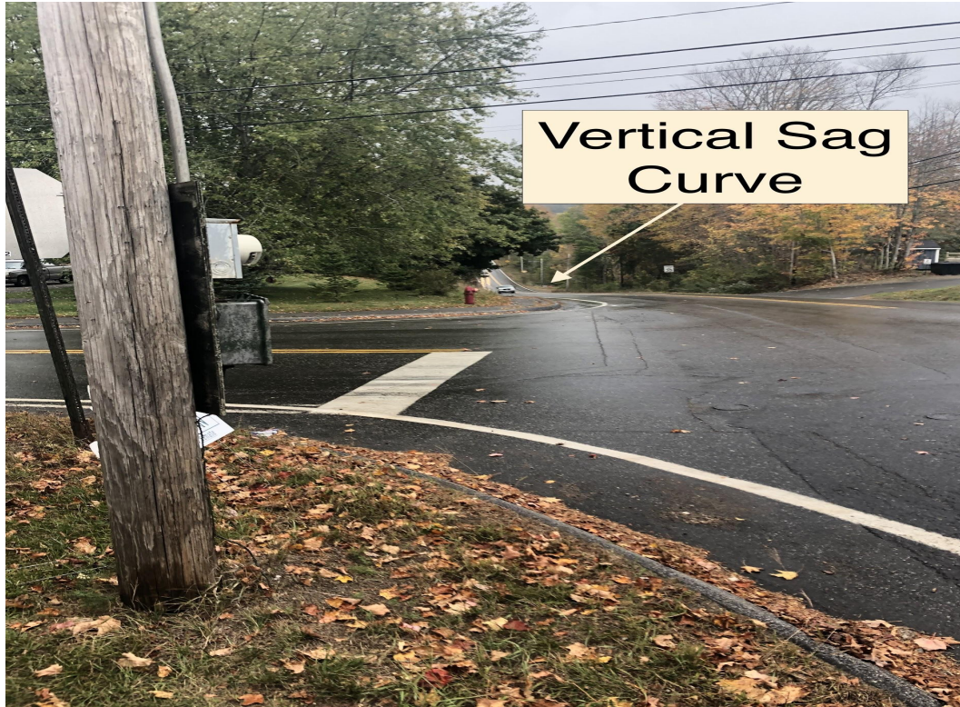
Figure 3.2 Shows the Vertical Sag Curve from WB approach
