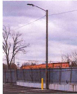
These lights can also be mounted on a wood utility pole.
