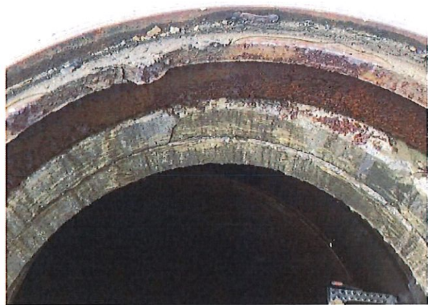
Manhole SMH007010: Infiltration in chimney, wall joints, and frame seal; cracking in chimney.
