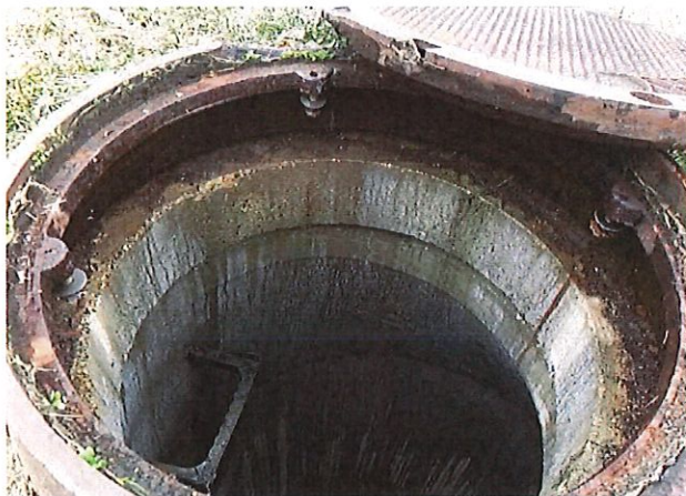
Manhole SMH105022: Broken frame and cover.
