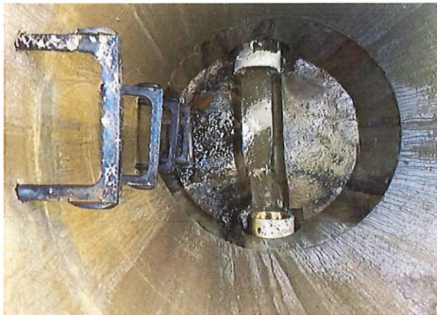
Manhole SMH006030: Infiltration in wall joints, infiltration in chimney, corroded frame.
