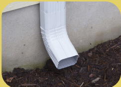
Gutters should not drain into sewers.
