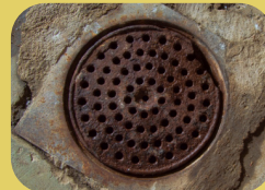
Basement drains must not go to sanitary sewers.
