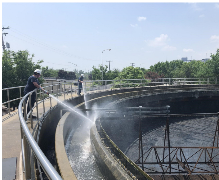
Maintenance of Secondary Clarifiers
