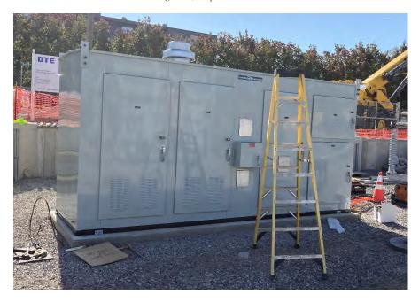
The last structure on the site is ITC's control center, which like DTE's PDC, encloses the equipment ITC uses to operate and protect their electrical equipment.
