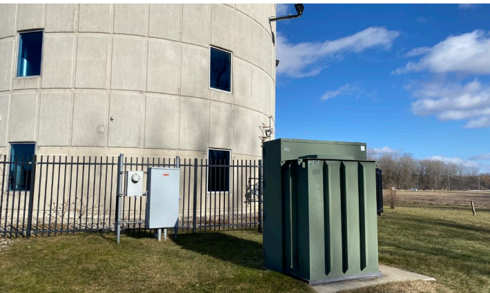
Transformer on concrete pad
