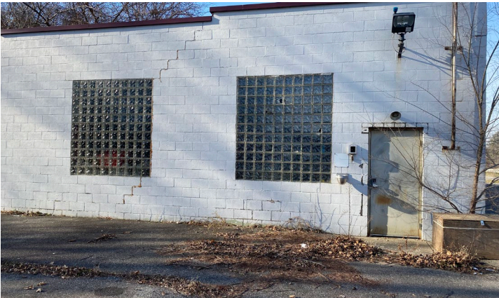
Glass block windows and side entry/exit door
