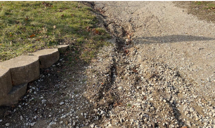
Hill erosion near boat house
