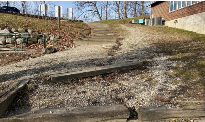
Hill erosion near boat house
