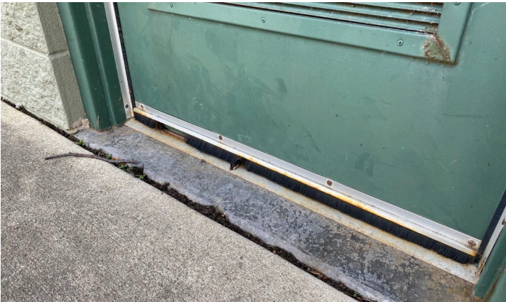
Restroom #1 door weather striping
