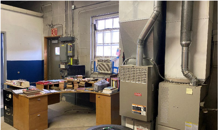
Gas fired forced air furnace
