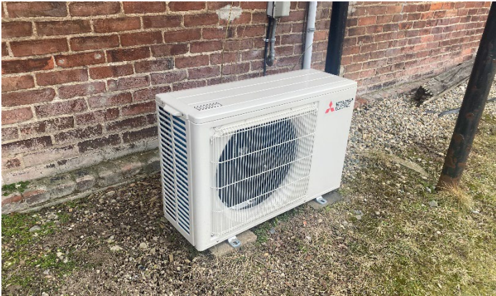
A/C condensing unit
