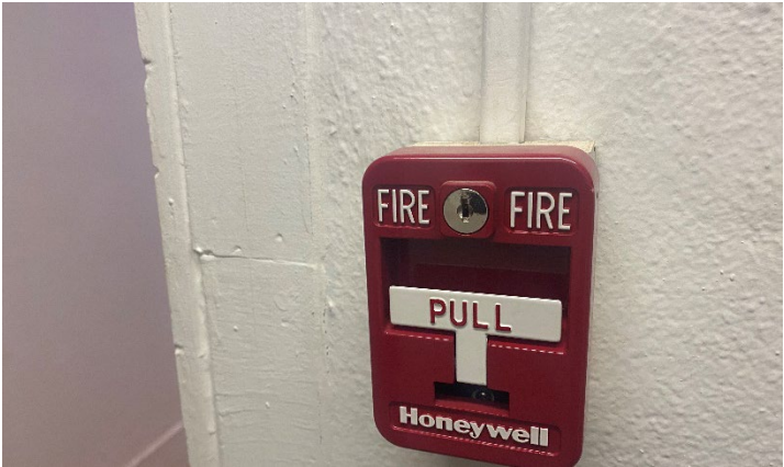
Fire alarm pull station
