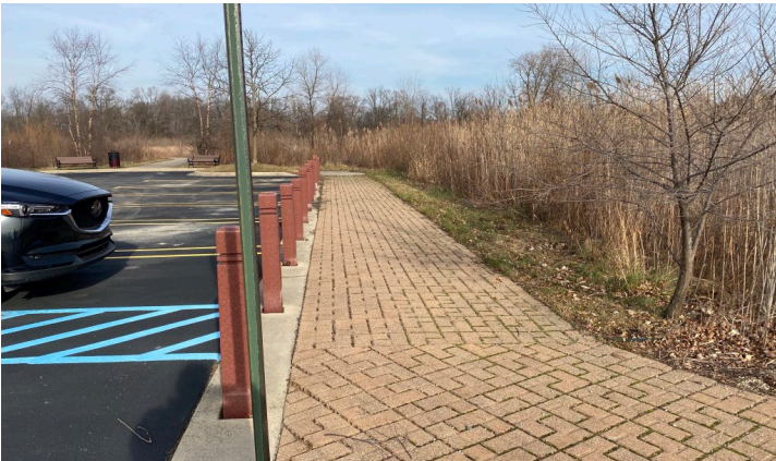
Brick paver sidewalk
