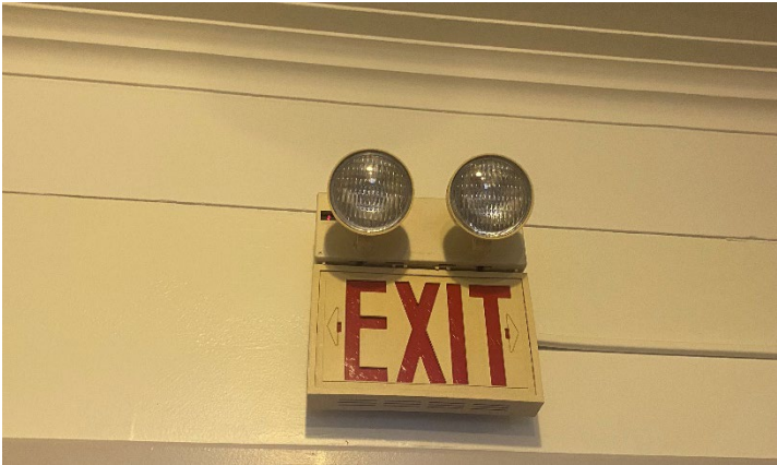
Exit sign and emergency lighting
