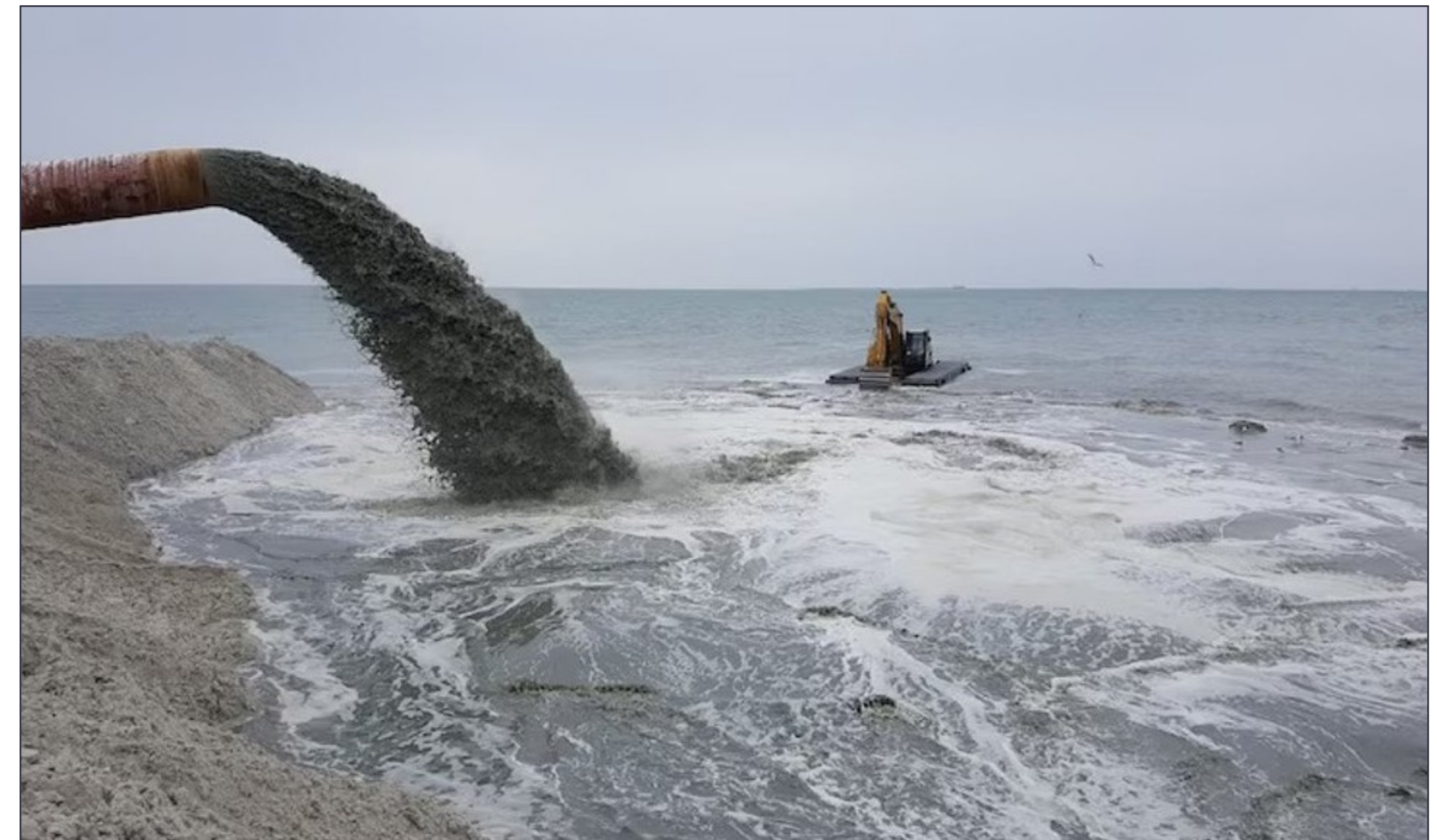
Figure 101. Rebuilding Coastline with Dredge Material (Photo Source: USACE)
