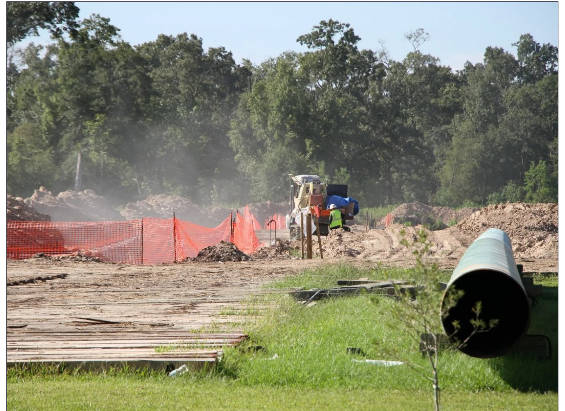
Figure 98. New Pipelines in Liberty County (Photo Source – Bluebonnet News)
