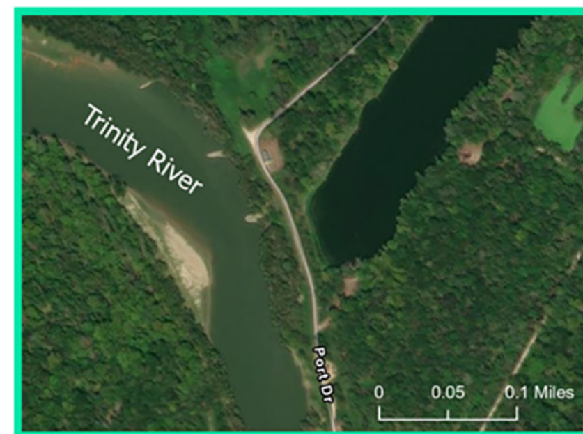
Trinity River channel narrowing caused by sedimentation near the northern end of the oxbow, along the west side of the Trinity River.
