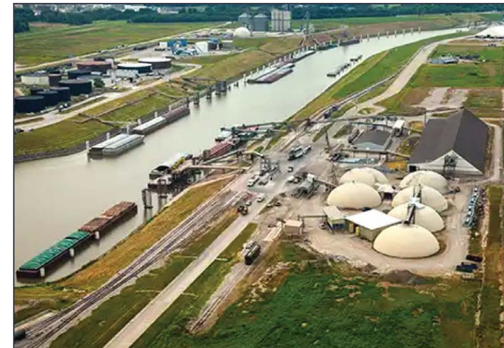
Dry bulk terminal (Tulsa Ports website)
