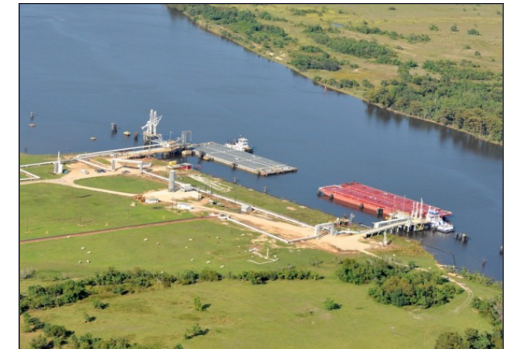
Neches River Barge Dock (Lanier Engineers website)
