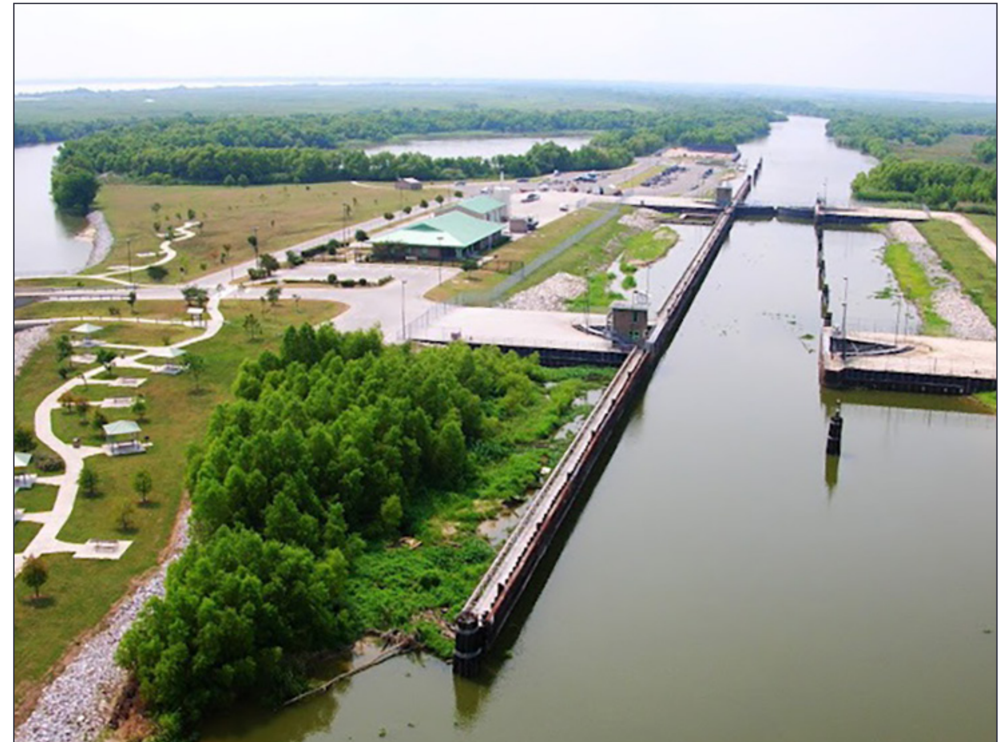
Figure 20. USACE Wallisville Lake Project
