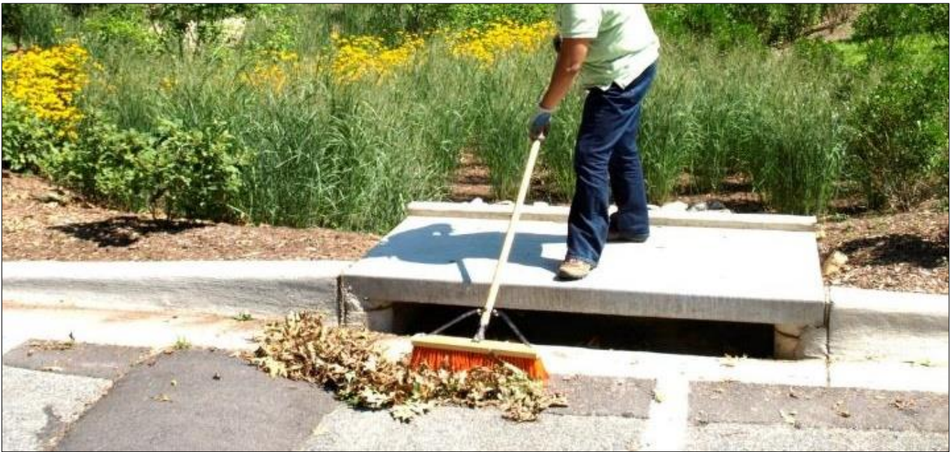
Move organic debris back onto lawns or into compost piles to avoid storm drain clogs and impacts to aquatic health in local streams (credit: www.mvareenmontaomerv.com ).
