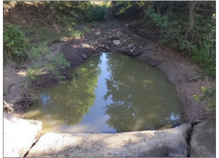
Example of a site with some impacts from illegal dumping.
