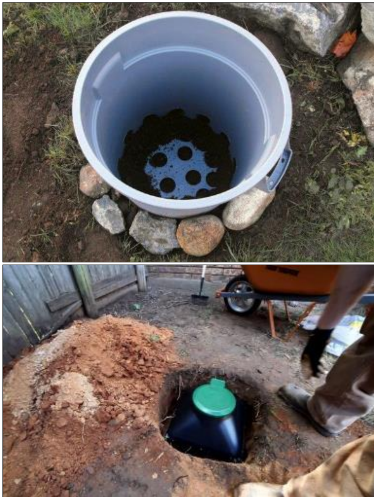
Above: Installation of DIY pet waste digester (Zach Ogilvie, www.instructables.com ). Below: Installation of prefabricated pet waste digester near Lake Arlington.
