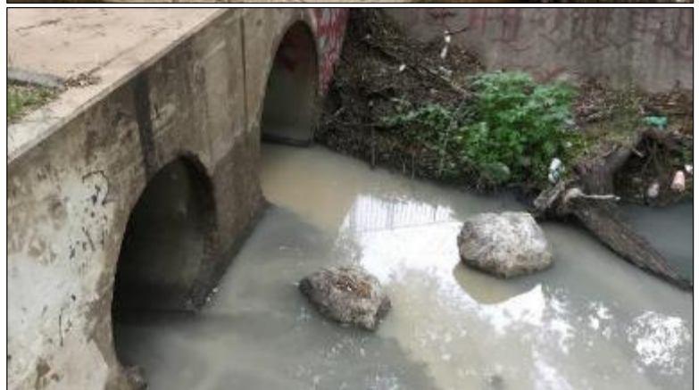
Above: Active SSO with flow from sewer access (credit: City of Arlington). Middle: Evidence of recent wet-weather SSO – note debris around rim (credit: City of Fort Worth). Below: Underground SSO, emerging at a culvert (credit: City of Fort Worth).
