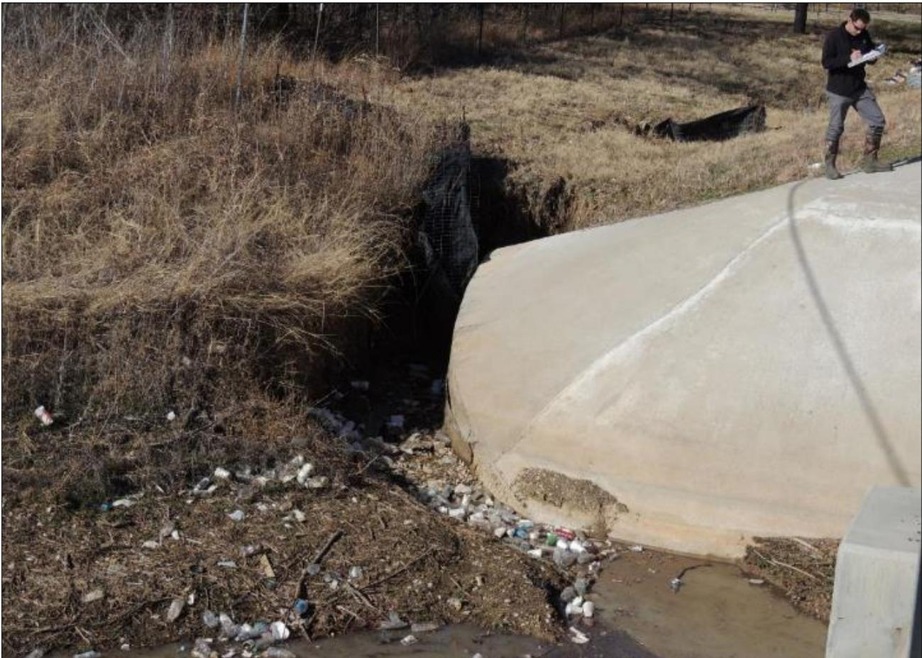
Survey site on Wildcat Branch impacted by both floatable trash and significant erosion.
