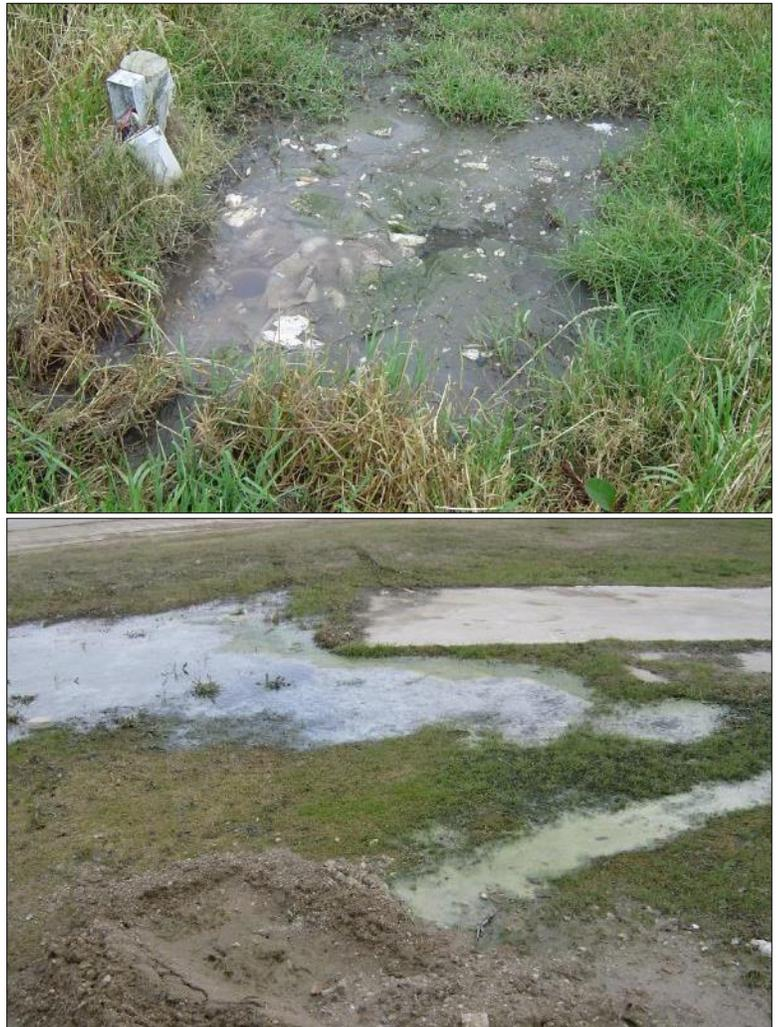
*OSSF malfunctions can occur due to lack of maintenance, improper construction in unsuitable soils, or overloading the drain field, resulting in overflows at the surface (City of Arlington).*
