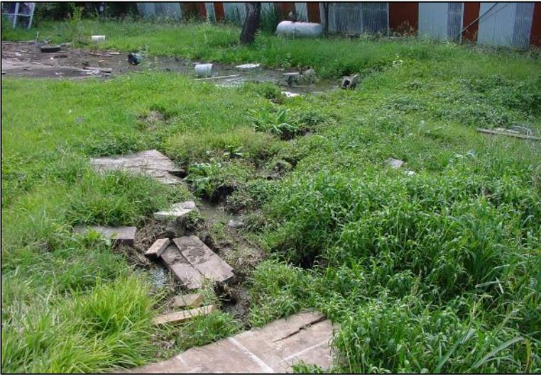
Pooled effluent seeping from malfunctioning OSSF (credit: City of Arlington).
