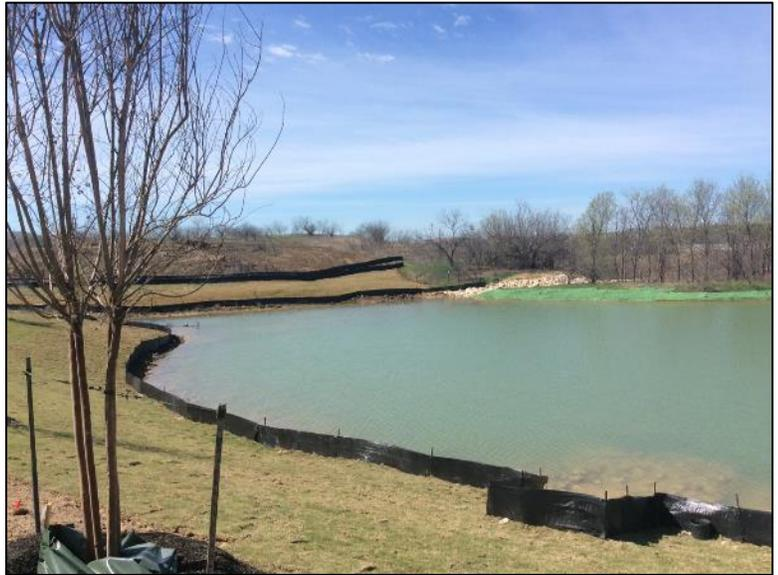
*Construction BMPs for stormwater pollution (silt fences, green curlex mat, sod replacement) near a development's retention pond (credit: City of Fort Worth).*
