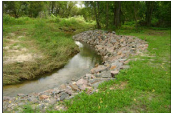
Riprap installed on an eroding streambank.
