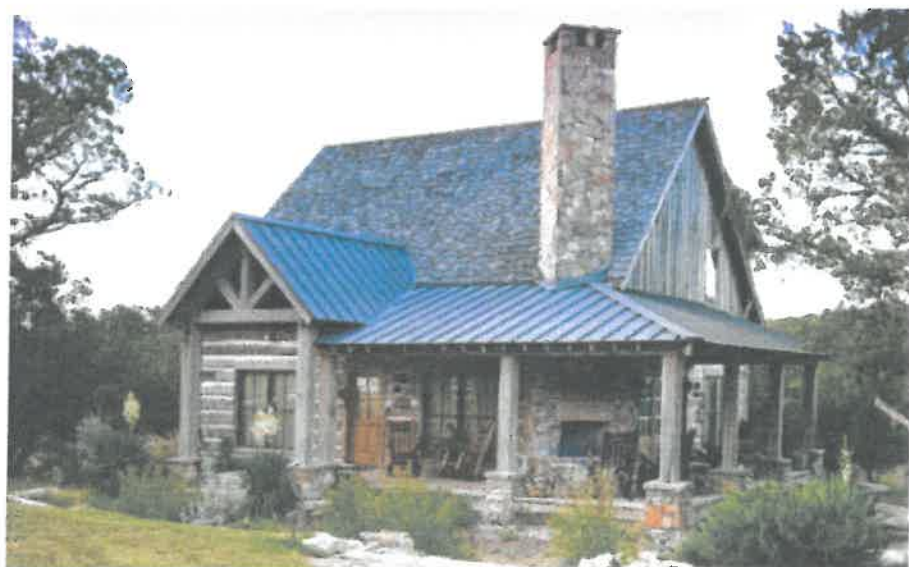
EXAMPLE OF "TIEING IN" METAL ROOF TO SHINGLE ROOF; ROOF SITS ON MAIN HOUSE JOIST
