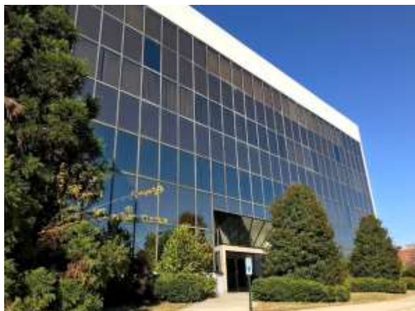
Photo 8: Vacant Corporate Office Space Near Downtown
