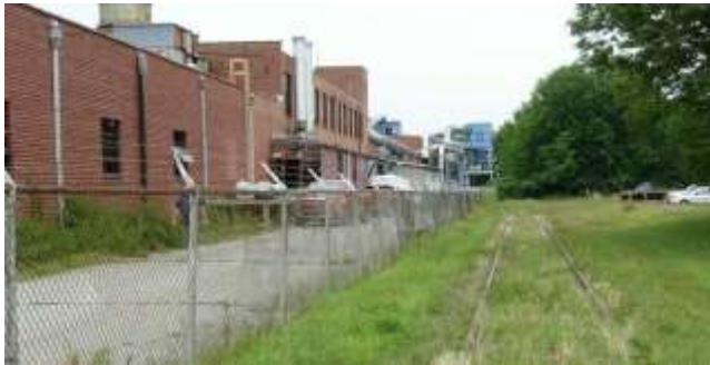
Photo 16: Old Industrial Property and Abandoned Rail Line
