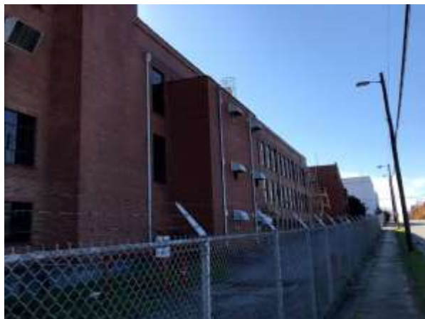
Photo 9: Old Manufacturing Buildings in Need of Brownfield Assessment and Clean-up
