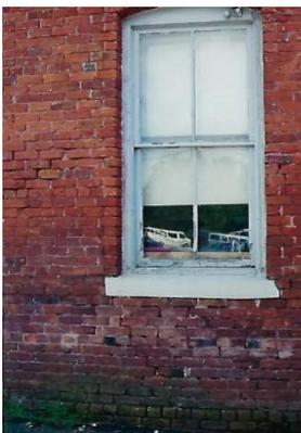
*This photo shows open masonry joints below and to the left of the window in need of repointing.*
