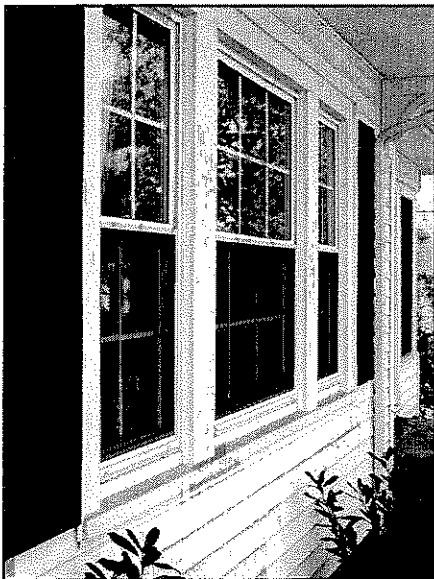
These operable doublehung storm windows match the existing windows in overall configuration and color, minimizing their appearance.
