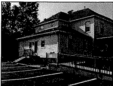
This one story addition is inset from the corners of the rear elevation and is compatible in terms of massing, materials, roof form, and windows with the original building.
