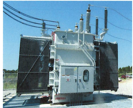
Figure 6. GSU Transformer with Secondary Containment to Capture any Leaked Oil
