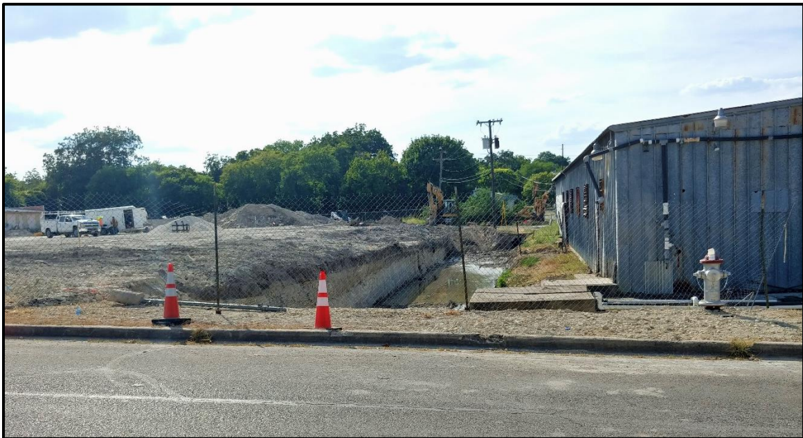
Drainage channel between lots, facing west from N. 1 st St,
