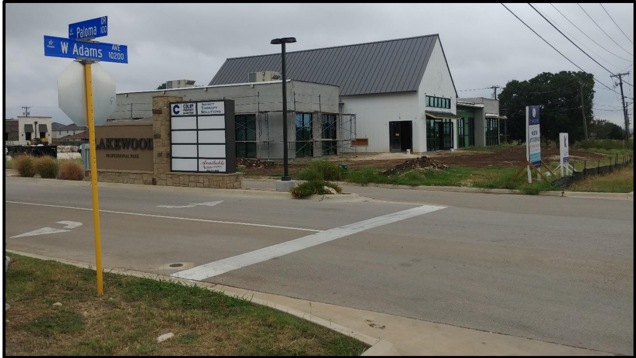
Facing east from intersection of W Adams and Paloma Drive
