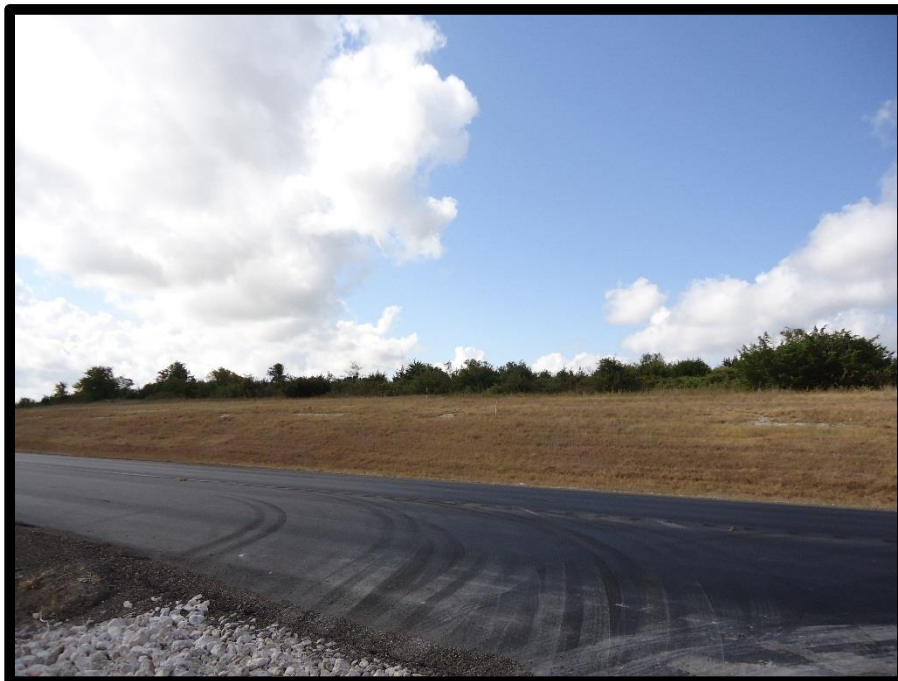
South: Undeveloped – Looking across Loop 363 (C & LI)
