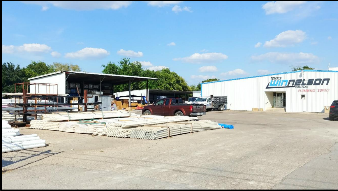
Existing warehouse, facing east from N 3 rd St
