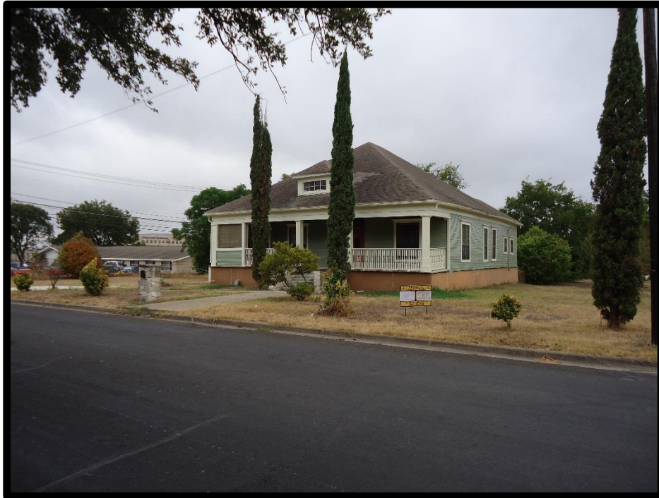
Site: Existing (unoccupied) SF Residence from W. Ave R (2F)
