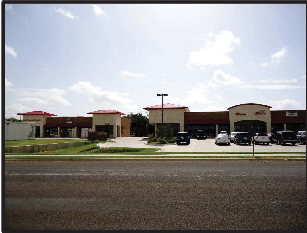
Site: Paint Brush Plaza (From Ermine Trail) (C)
