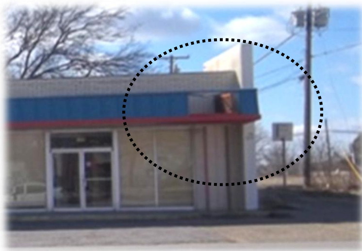
Current canopy damage on far west side of Central Ave. building elevation.
