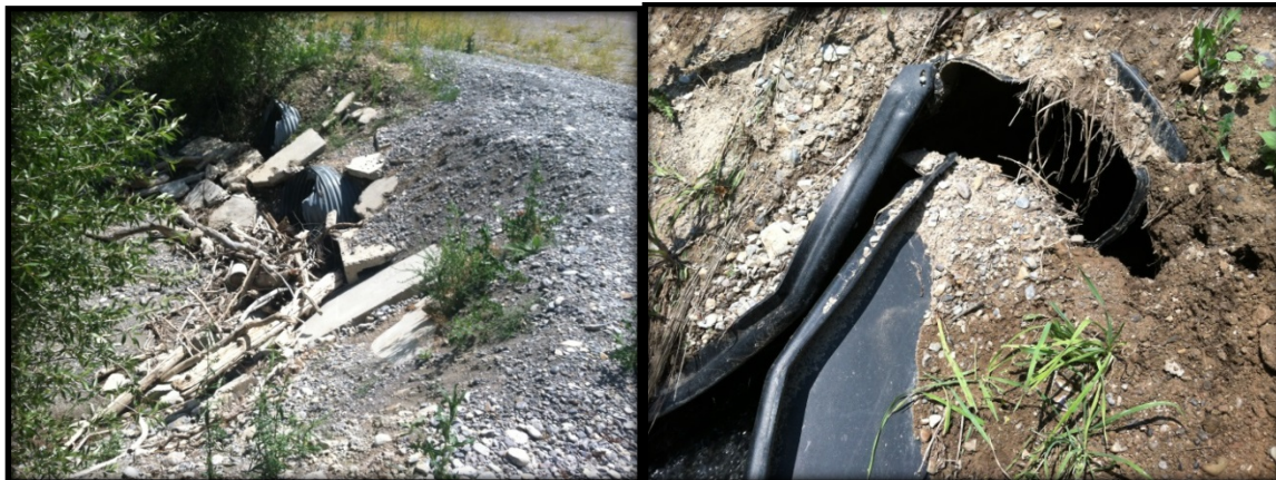
Woody debris at Cedar Creek and Runway & Collapsing flare end treatment
