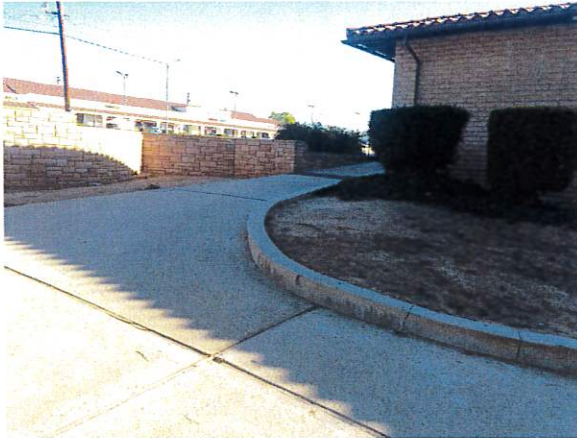
BEFORE, non-ADA compliant sloping ramp
