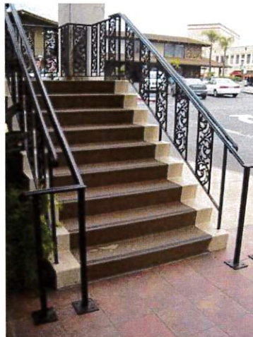
New ADA, stair nosing and handrails
