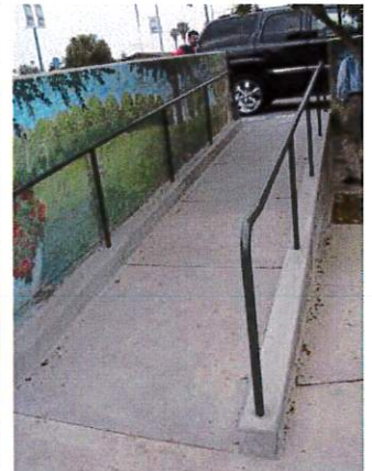
New ADA, stair nosing and handrails at parking structure
