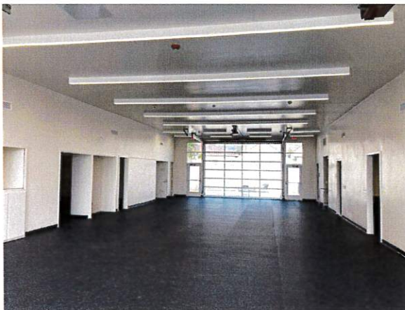
New Rubber Sports Flooring wall finishes, LED Lighting
