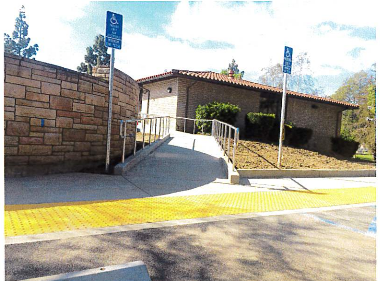
AFTER, new ADA compliant entry ramp
