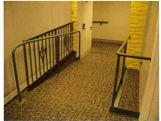
New ADA Compliance improvements at the Civic Center entry reception counter, public restrooms, interior ramp with new handrails
