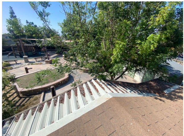
Debris build-up on front awning
