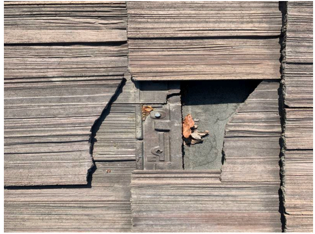
Broken concrete tile on Community Center Building
