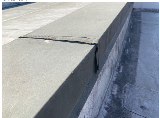
Weathering at coping cap laps
