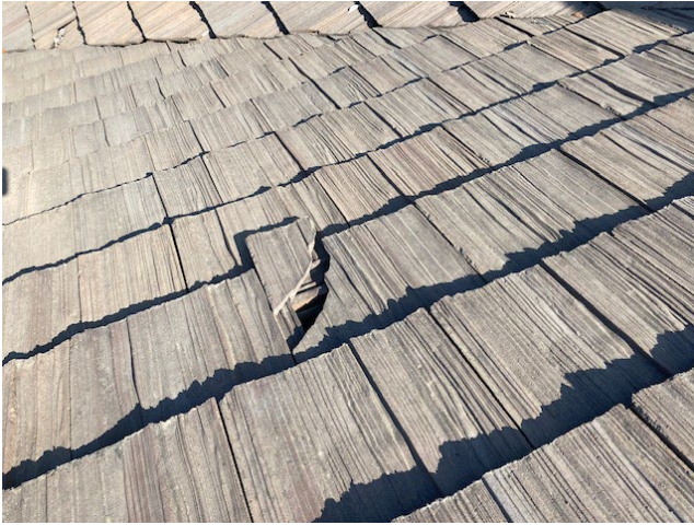
Broken concrete tile on Restroom Building
