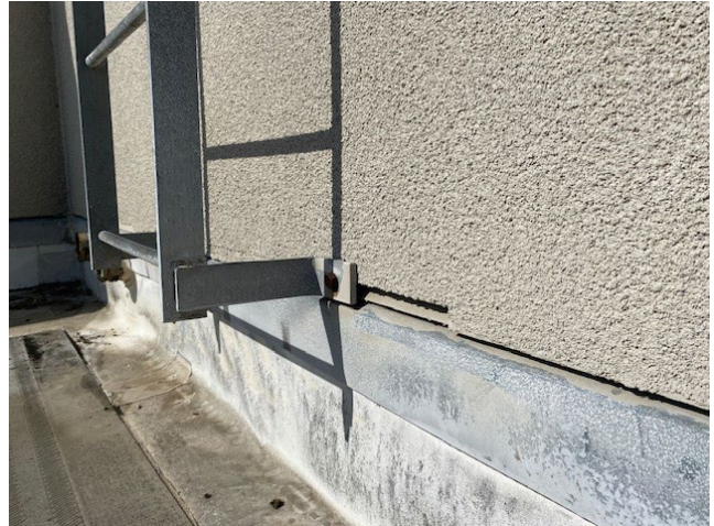
Spalling stucco at reglet
