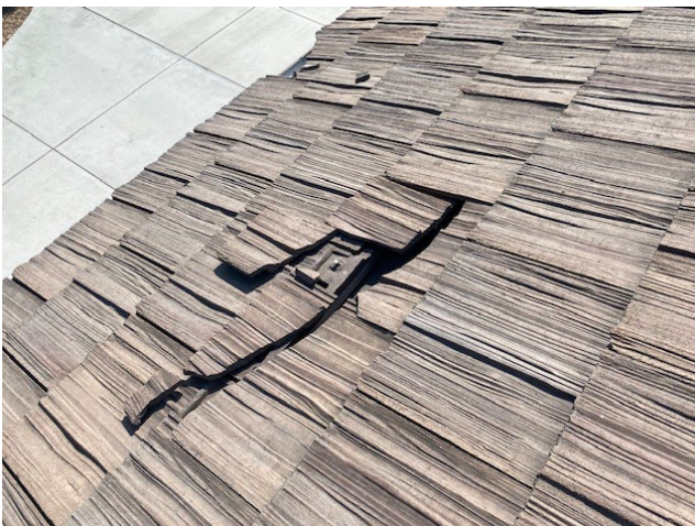
Broken concrete tile on Restroom Building
