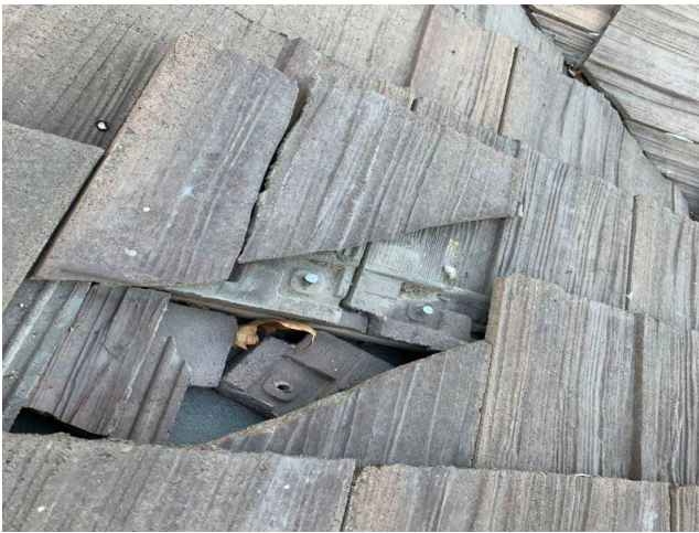
Broken concrete tile on Community Center Building
