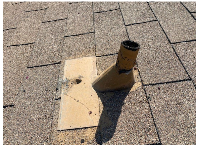
Sealant Failure at Penetration Flashing
