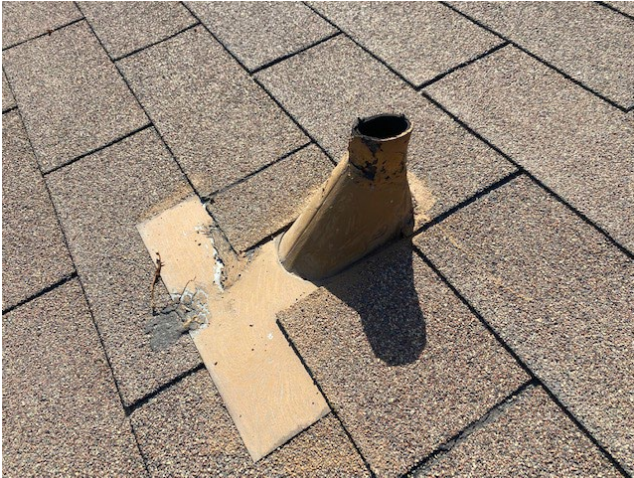
Sealant Failure at Penetration Flashings
