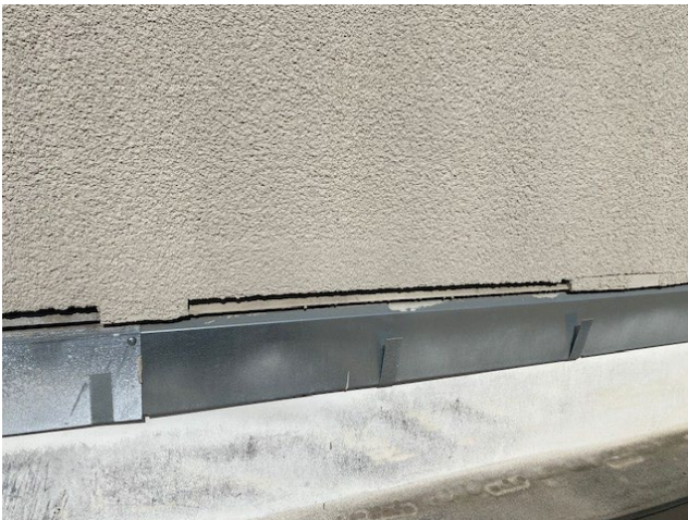
Spalling stucco at reglet
