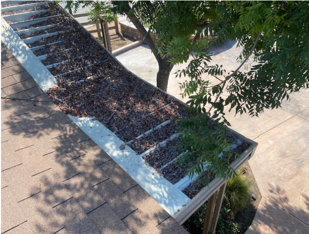
Debris build-up on front awning
