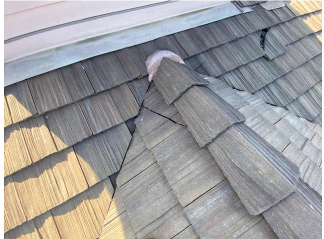
Broken concrete tile on Restroom Building
