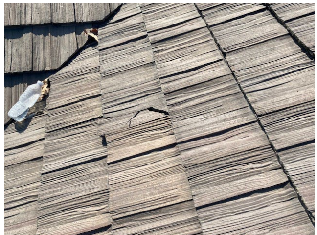
Broken concrete tile on Restroom Building
