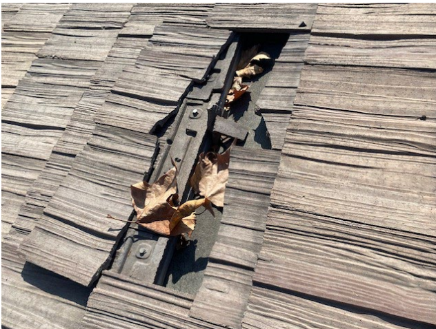
Broken concrete tile on Restroom Building
