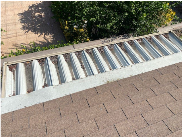
Debris build-up on rear awning
