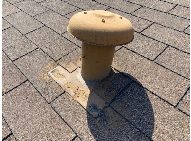
Sealant Failure at Penetration Flashings
