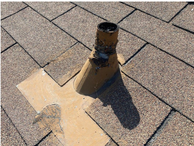
Sealant Failure at Penetration Flashing
