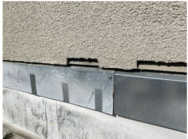
Spalling stucco at reglet
