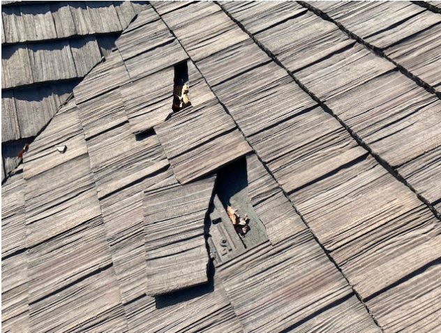
Broken concrete tile on Restroom Building
