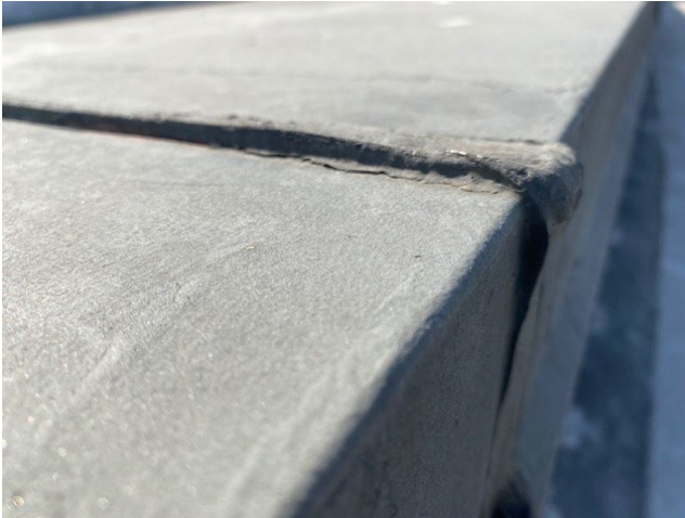
Weathering at coping cap laps
