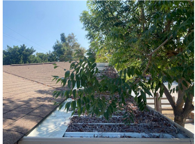
Debris build-up on front awning
