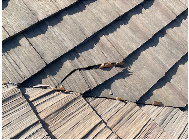
Broken concrete tile on Restroom Building
