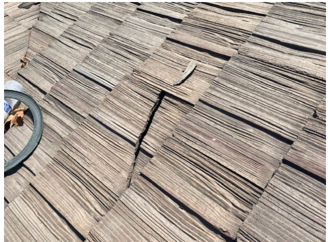
Broken concrete t tile on Restroom Building
