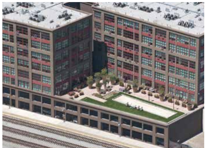
Podium building featuring a two-story parking garage on lower levels
