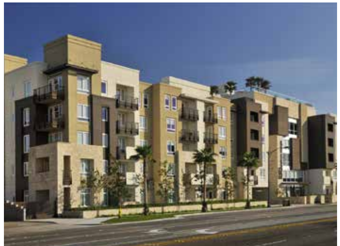
Five-story podium structure includes parking on lower stories with dwelling units located above.
