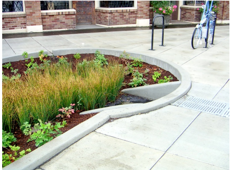
Rain gardens and bioswales help capture and filter stormwater, recharging our aquifers and improving the quality of our waterways.
