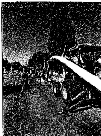
HDPE allowed the city of Covina to install a new pipeline without disruption of important community areas like a hospital, baseball field, neighborhoods, and trailer park.
