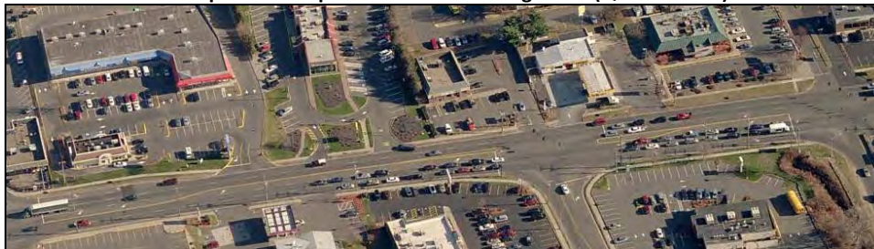
Example Of Multiple Curb Cuts And Congestion (Queen Street)
