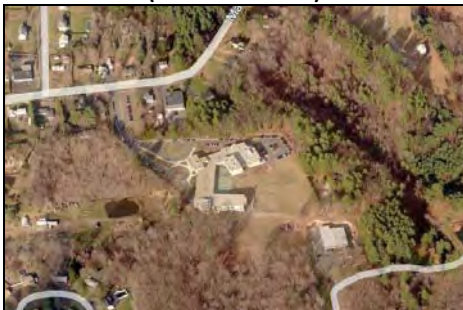
Strong Elementary School (Southwest Area)
