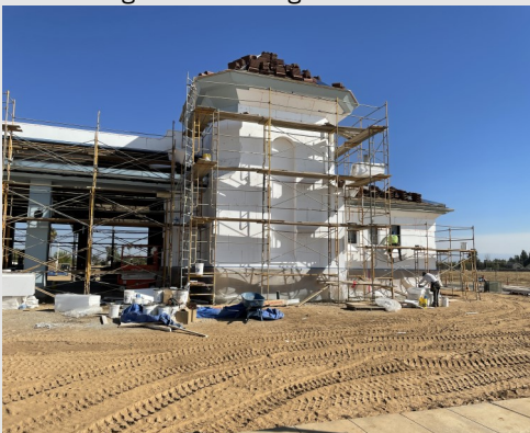
EIFS System install begins
