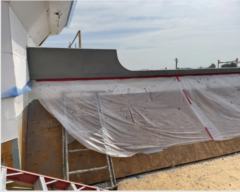
Plaster work at high roof has begun
