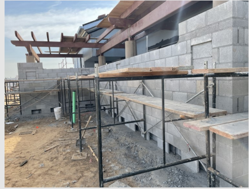
CMU block fence being constructed
