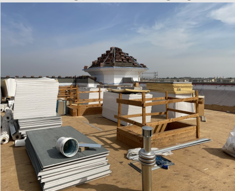
Roofing Material being loaded on Roof
