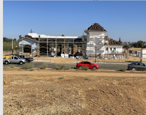
North facing view of Fire Station
