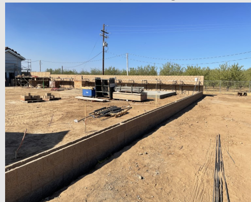
Perimeter CMU fence being constructed
