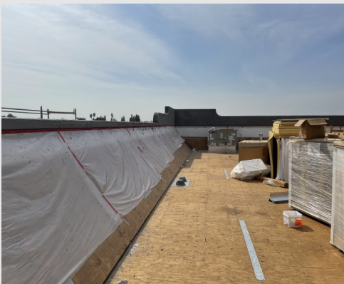
Roofing preparation is ongoing
