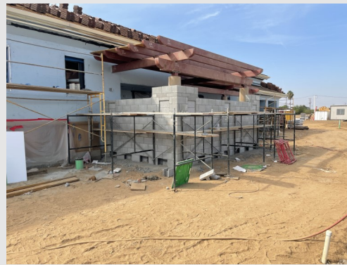
CMU block fence at patio being constructed
