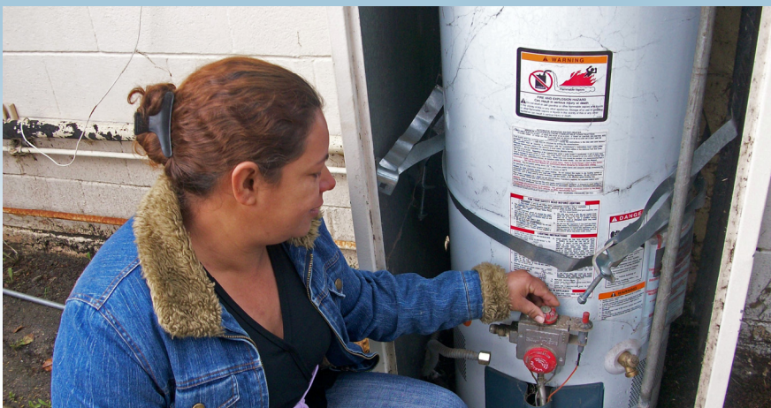
Housing Authority resident and employee Maria Calix installs a new energy efficient water heater. Maria was a graduate of the Green Construction training program.
