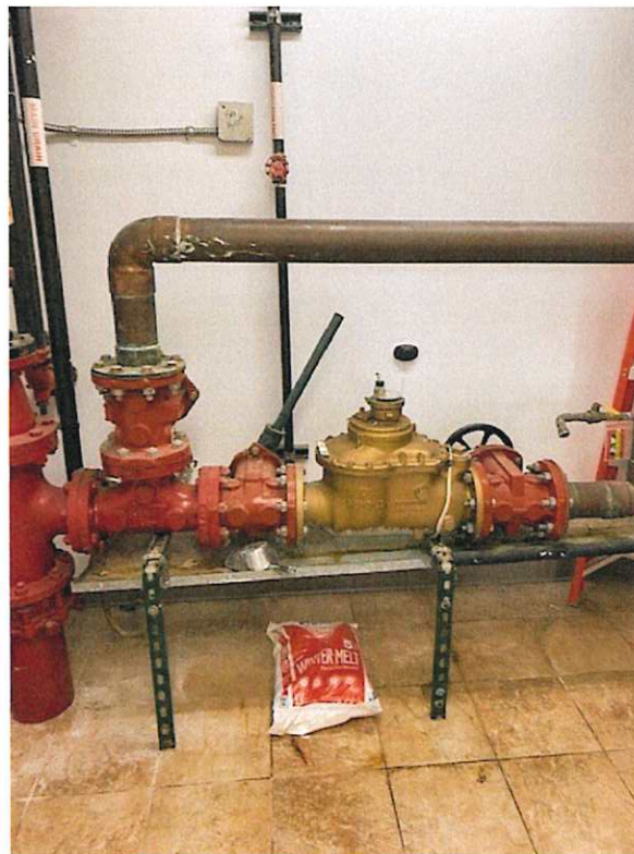
PHOTOGRAPH 4: Existing Water Meter at The Brooks Assisted Living.
