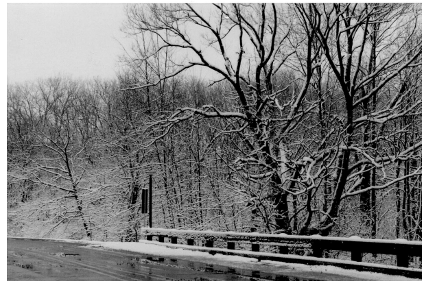
The old, wooden bridge over Paint Creek
