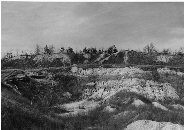
Early photo of the brick yard excavations
