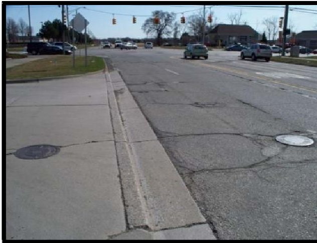
Eastbound approach along Auburn Road
