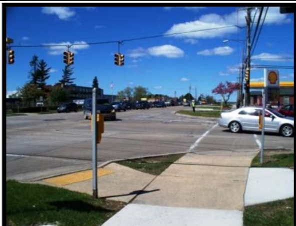
Tight turn radius from southbound Rochester Road to eastbound Avon Road.
