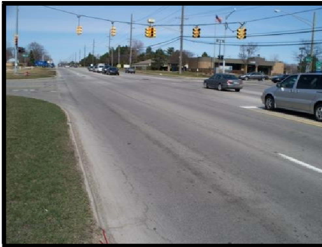
Northbound approach along Rochester Road
