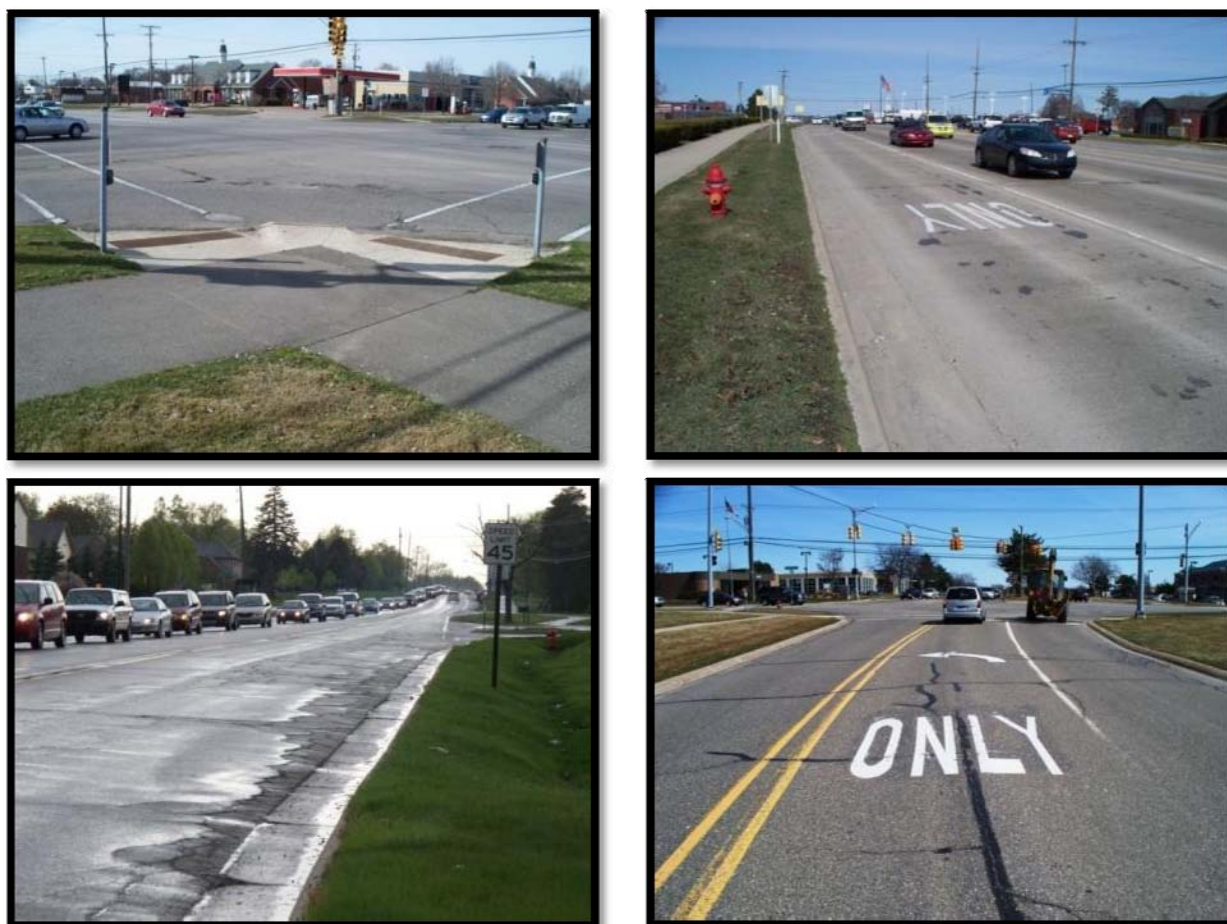
Figure 3-1 CURRENT CORRIDOR CONDITIONS
