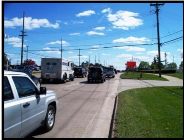
Poor signal visibility as a result of the crest vertical curve on the eastbound approach of Avon Road.
