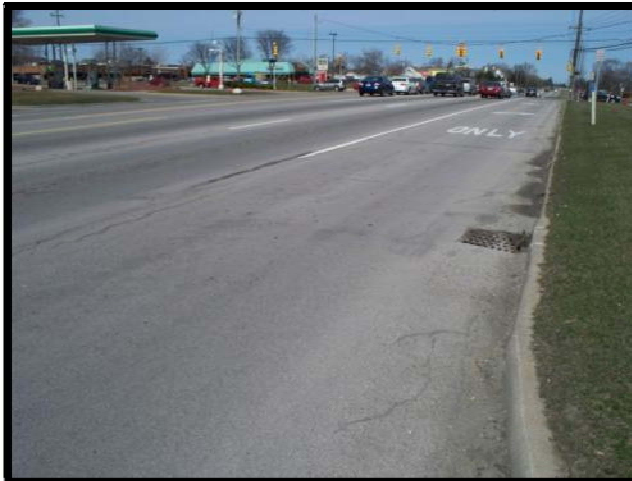
Northbound approach along Rochester Road
