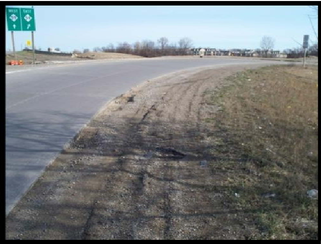
Eastbound M-59 entrance ramp
