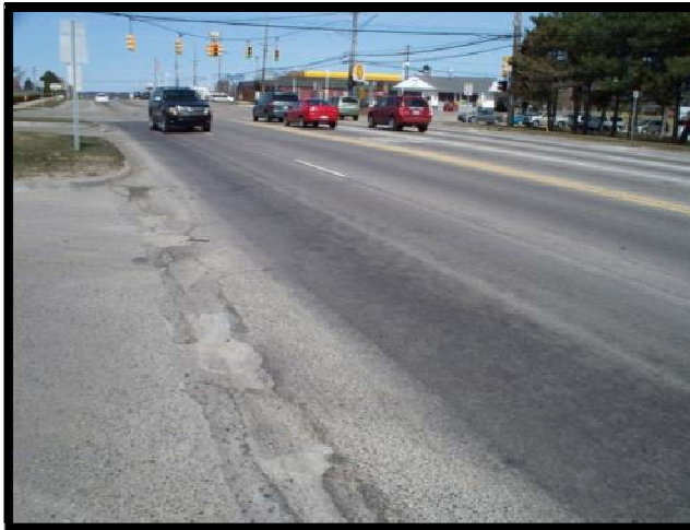
Northbound approach along Rochester Road
