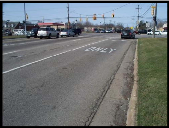
Westbound approach along Auburn Road
