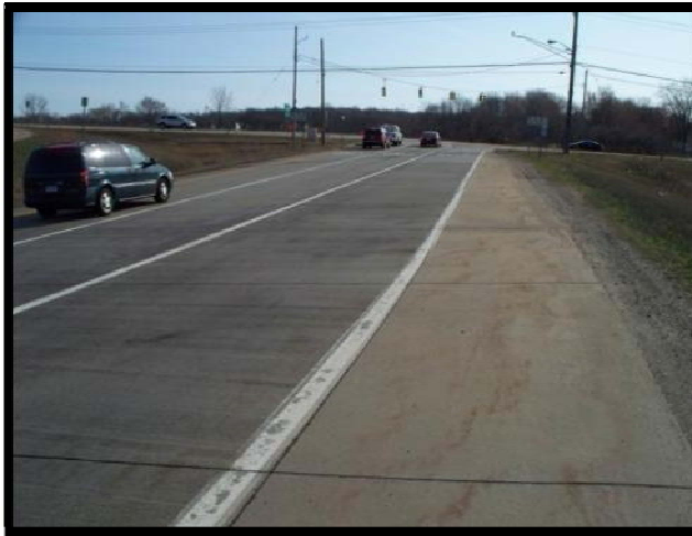
Eastbound M-59 exit ramp
