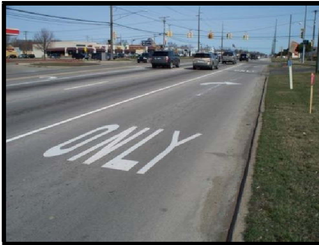
Northbound approach along Rochester Road
