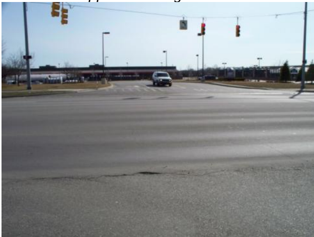
Looking Eastbound Meijer Driveway (Signalized)
