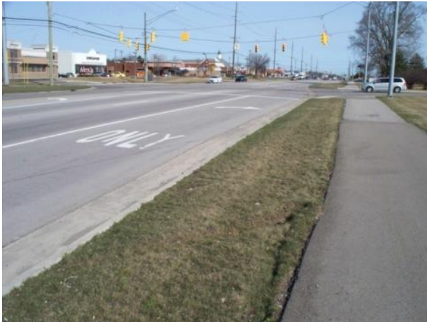
Northbound approach along Rochester Road
