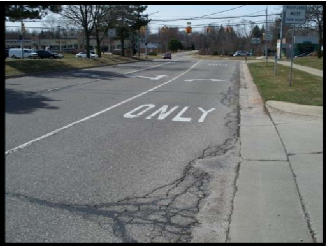
Westbound approach along Barclay Circle/Wabash Road
