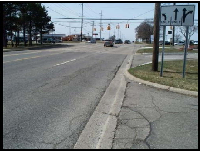
Westbound approach along Avon Road
