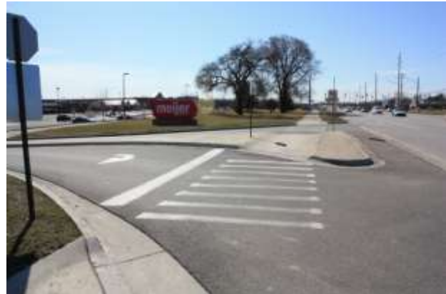
Example of Existing Access Management Application: Channelization of Access to Meijer shopping center
