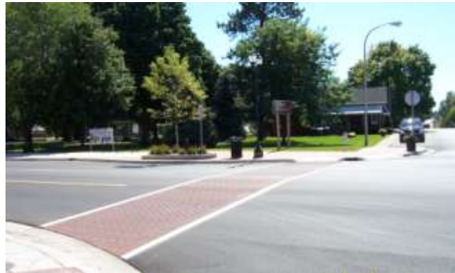
Example of how driveway design can draw attention to pedestrians in the crosswalk
