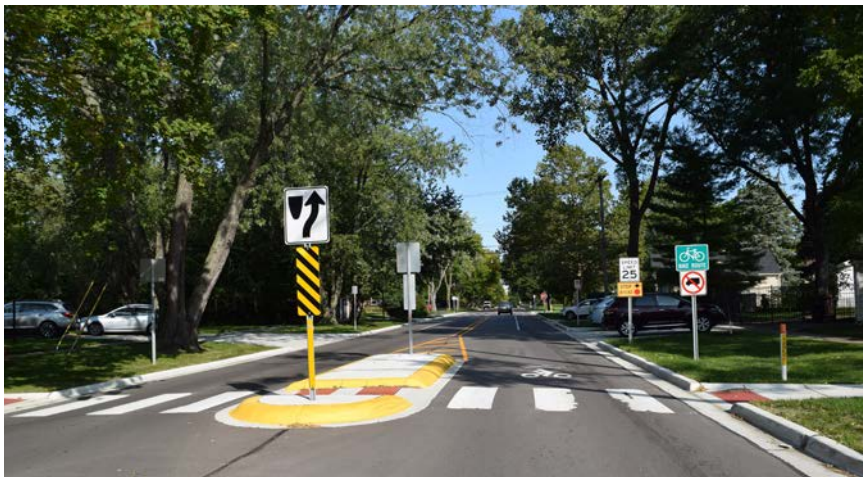
Mid-block crossing with pedestrian bicycle signage on Normandy Road in Royal Oak, MI.
