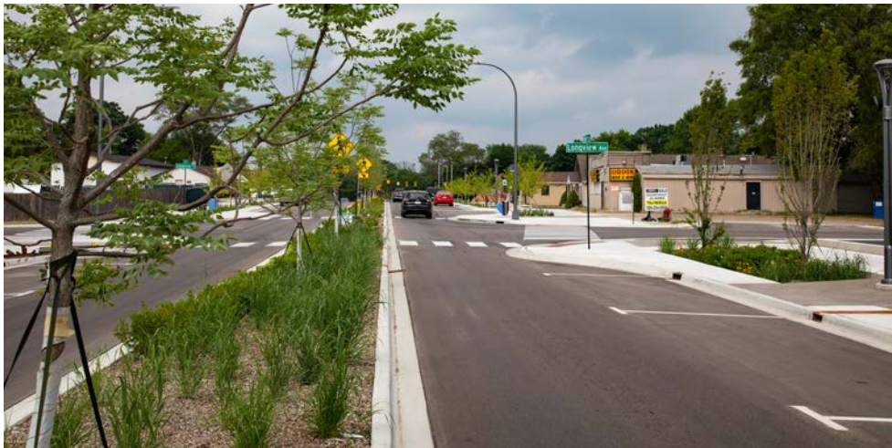
Access Management implementation on Auburn Rd via planted center median and streetscaping.
