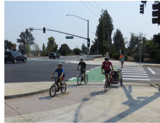
Key features include a corner island, forward bicycle queuing area, driver yield zone and pedestrian refuge median. Source: MnDOT Bicycle Facility Design Manual
