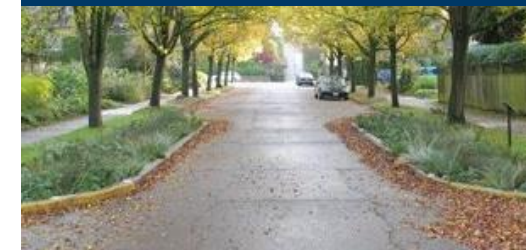
Pinchpoints narrow a street to one lane, drivers slow down and yield to other drivers. Seattle WA
