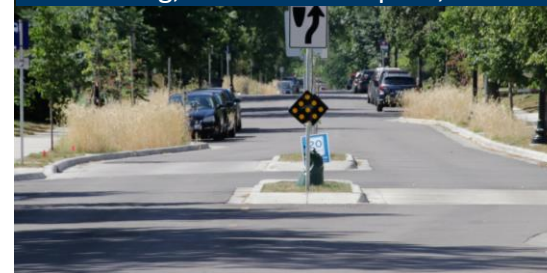
Chicanes are curb extensions that create a serpentine, horizontal shifting, effect. Minneapolis, MN
