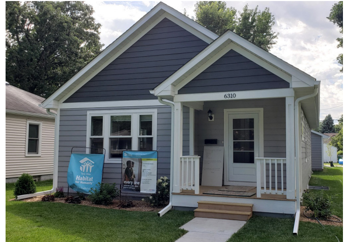
Richfield's partnership with Habitat for Humanity constructs affordable housing units in the city. All of their houses are built to meet Energy Star 3.1 standards.
