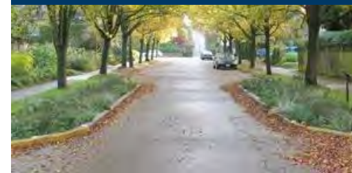
Pinchpoints narrow a street to one lane, drivers slow down and yield to other drivers. Seattle WA
