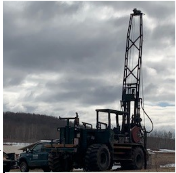
Geotechnical Drilling near Highbridge along the proposed Line 5 Reroute path
